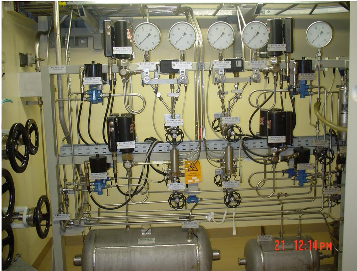
Figure 04.04-4-17: Picture of a Typical AMS Nitrogen System
