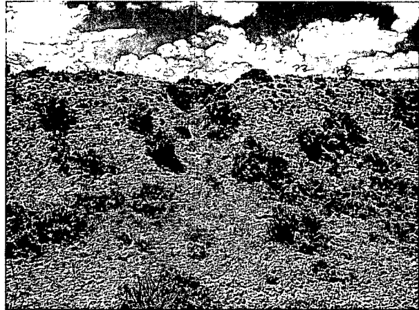
Photographs 7a & 7b. West channel bank, example of local bank erosion/rilling, 2008 on left, 2007 on right.
