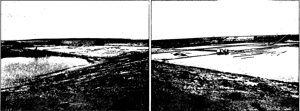
Photographs 3 and 4. Tailings surface from east embankment looking west.
