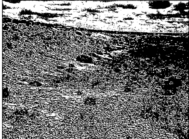
Photographs 8a & 8b. East channel bank, with local erosion caused by overland flow entering channel. Photographs taken in different locations in 2007 (right) and 2008 (left).
