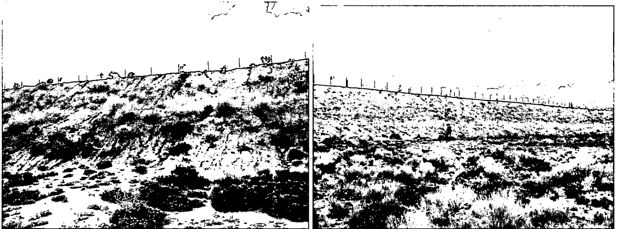
Photographs 12 and 13. Exterior of east and north embankments.
