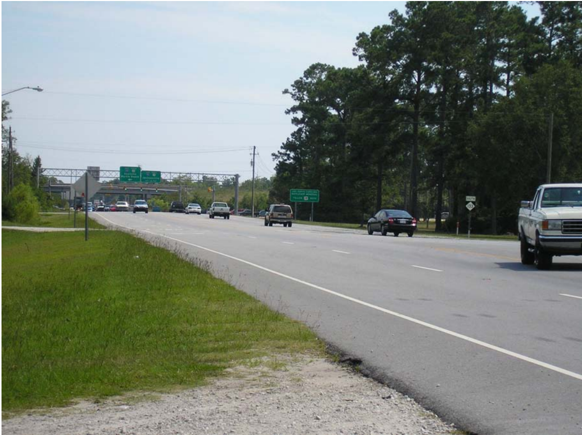
Figure 3.9-5. NC 133 (Castle Hayne Road), north of I-140.
