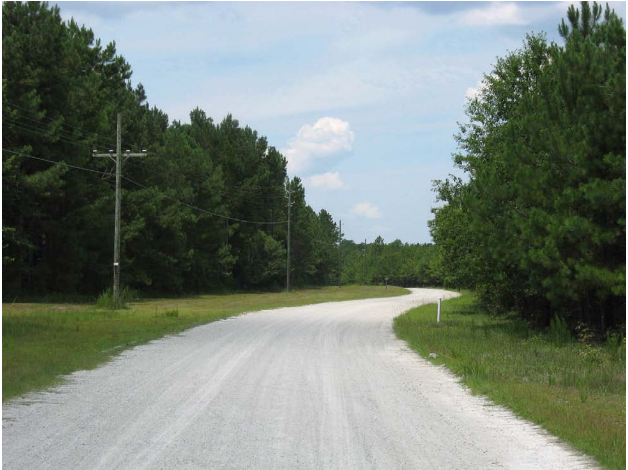
Figure 3.9-6. Power lines along an unpaved road on the Wilmington Site.
