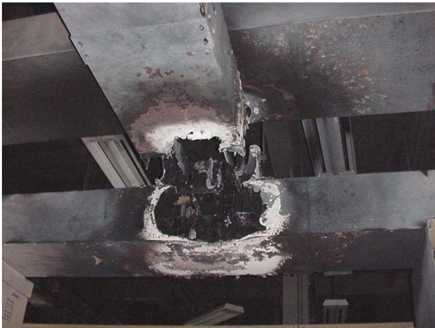
Figure 1: Photograph of the point on the bus duct where the arcing fault at Diablo Canyon was manifested (the fault point). Note that the tops of the cabinets to the left and right (the cabinets to the left are shown in figure 2) are visible in the lower corners of this photograph.
