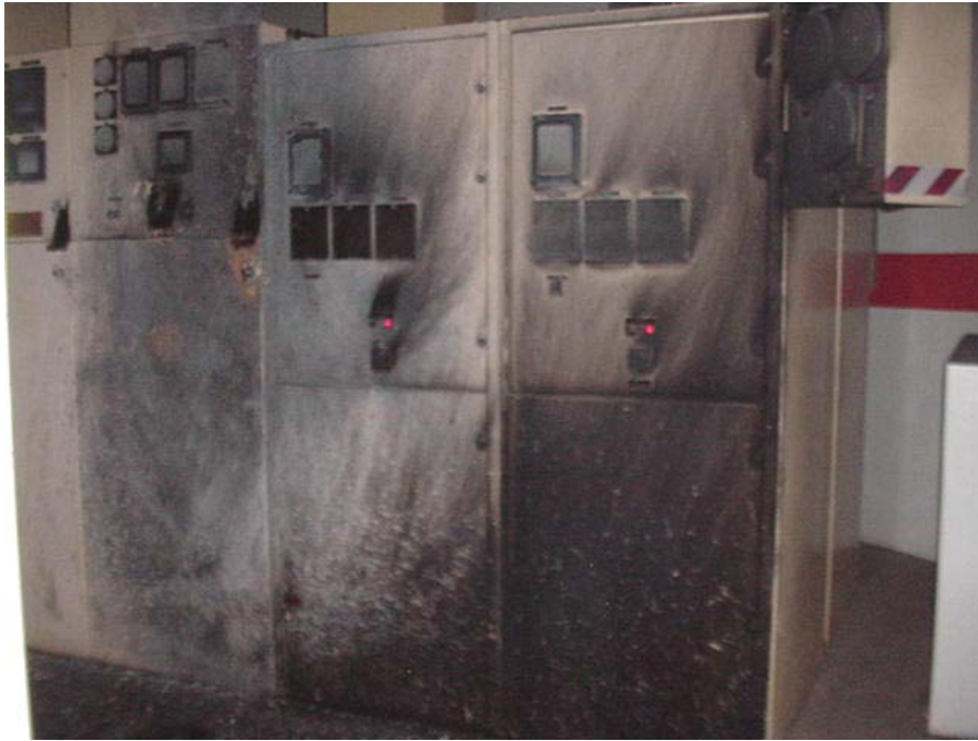
Figure 2: Photograph of the surface damage and burning observed for the more heavily impacted cabinets on one side of the aisle-way below the fault point (the cabinets to the left as seen in Figure 1).
