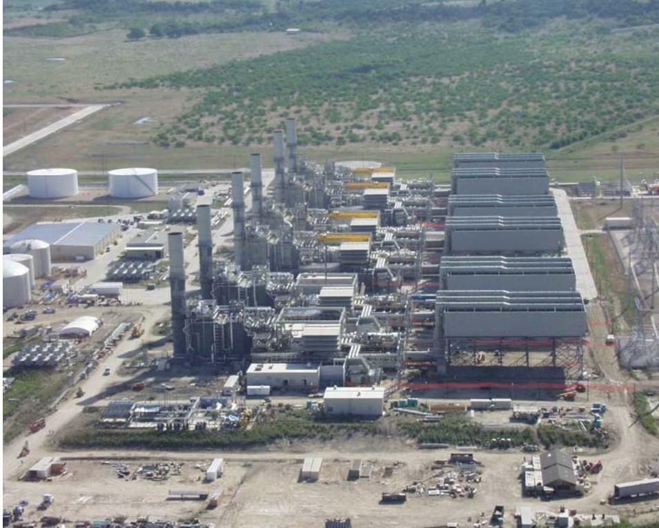
Photo 2: 4,000 MW Matimba dry-cooled coal-fired power plant in South Africa. Plant consists of six 665 MW units. The air-cooled condensers are in the foreground of the power plant.
