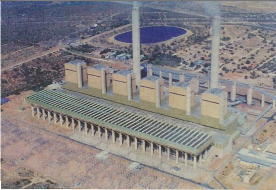
Photo 2: 4,000 MW Matimba dry-cooled coal-fired power plant in South Africa. Plant consists of six 665 MW units. The air-cooled condensers are in the foreground of the power plant.
