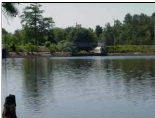
Figure 78. Glenville Lake at dam, Cumberland County.
