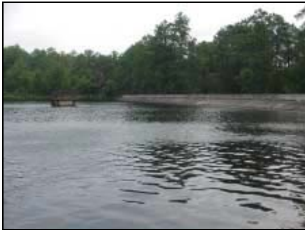
Figure 72. Old Town Reservoir, near the dam, Moore County.
