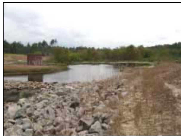
Figure 67. View from top of the dam of the “impoundment” near Nicks Creek at NC 22, Moore County.
