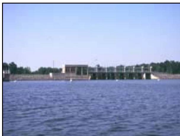
Figure 31. Dam at Cane Creek Reservoir, Orange County.
