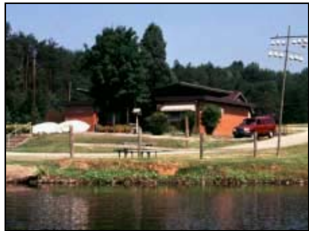
Figure 17. Park office at Lake Higgins, Guilford County.
