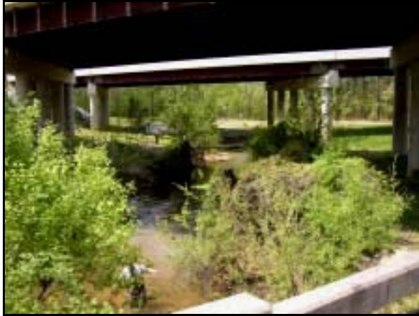
Upstream view of Little Alamance Creek at SR 3039, Guilford County.
