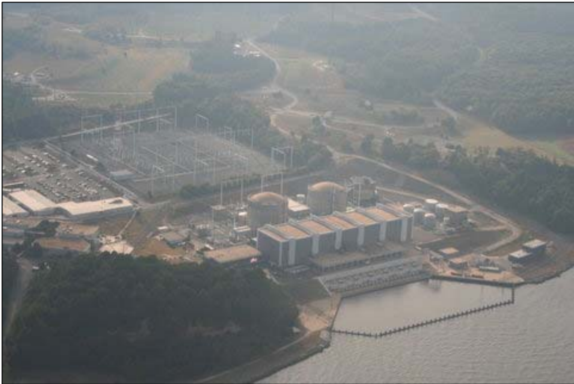
Calvert Cliffs Nuclear Power Plant - Photographer: John Swarey
