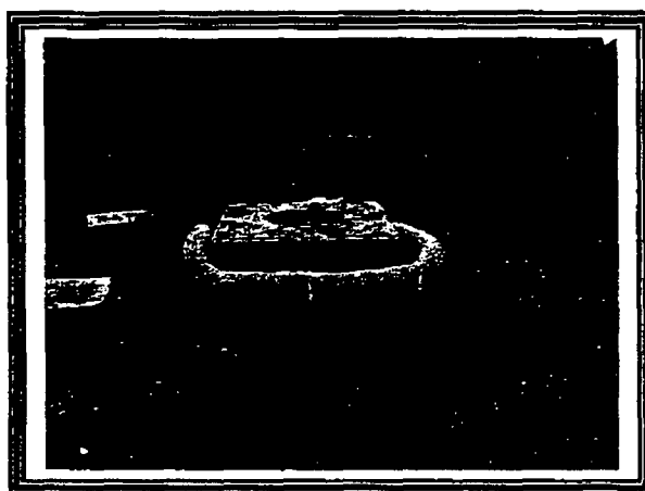
Sediment Tube Inlet Protection
