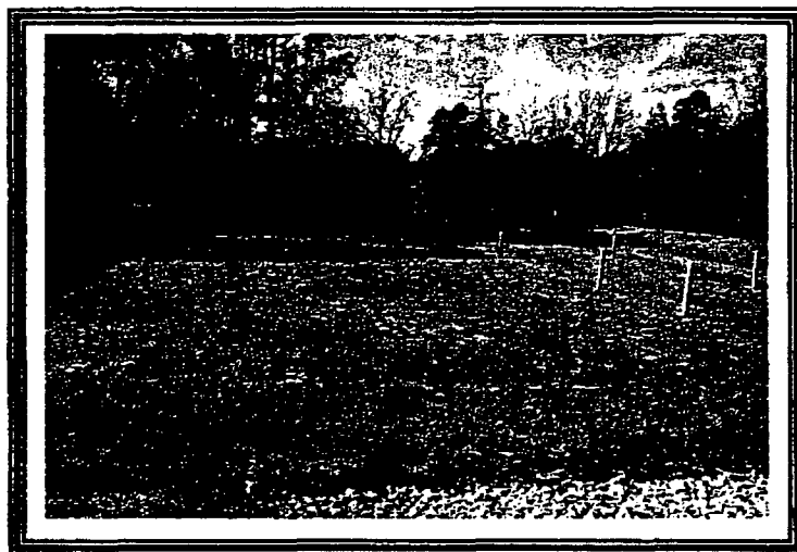
Bioretention Area with uncut clean outs
