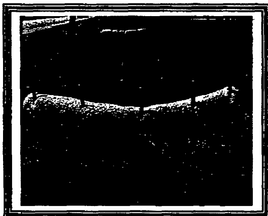
Sediment Tube Check Dam
