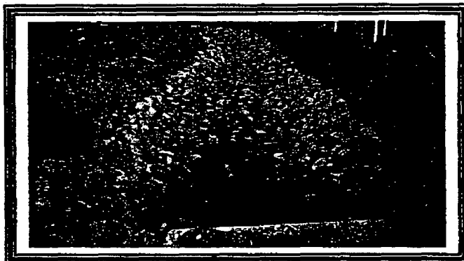
Riprap Lined Channel
