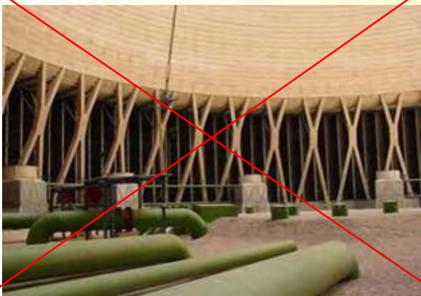
Dry Tower with delugable Peak Coolers (5-10%)
