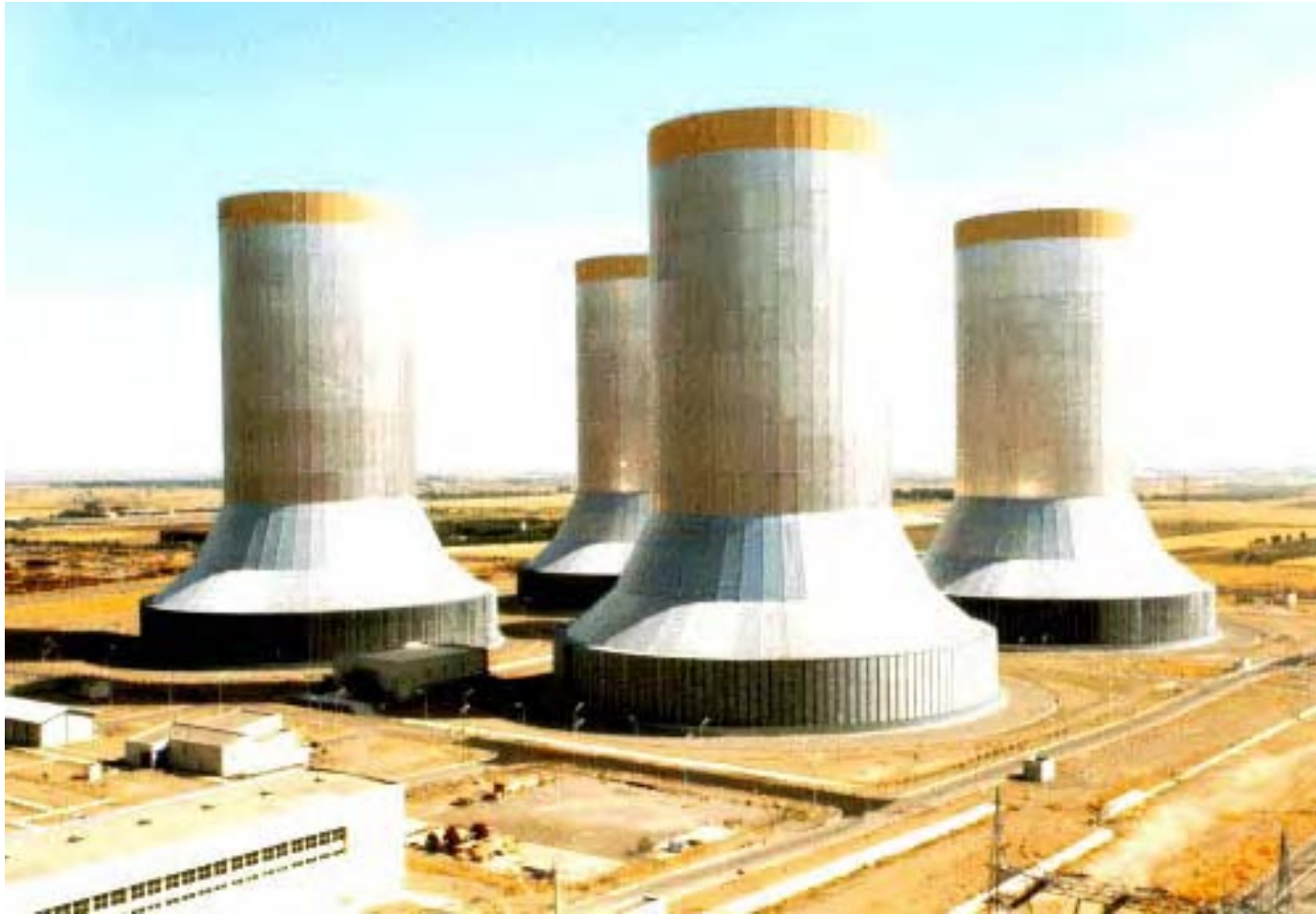
Natural Draft Cooling Towers at the Shahid Rajai TPP (4 x 250 MW e Iran) Turbine cycle: by MHI; Boiler: by IHI
