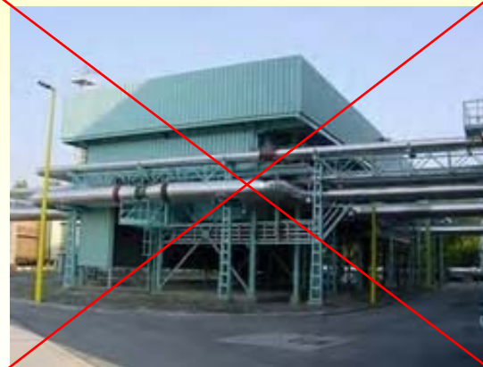
Dry/deluged Cooling System (10-35%)
