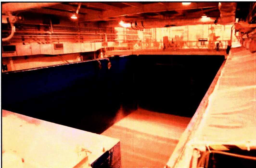
Figure 3-20. The Spent Fuel Pool After Deactivation
