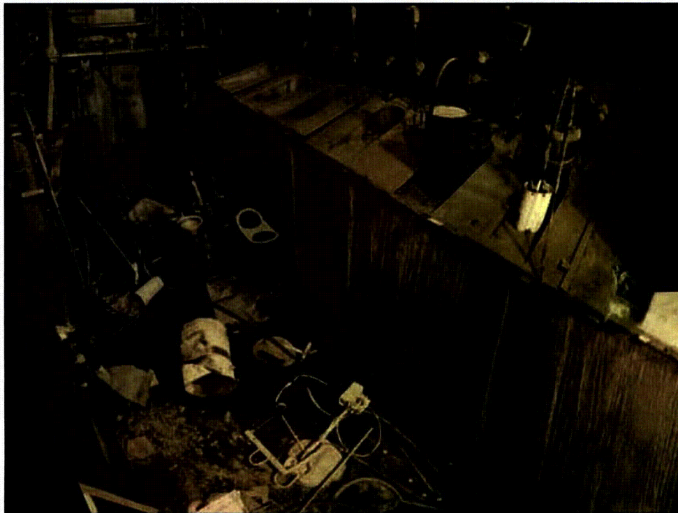
Figure 3-17. Conditions in the General Purpose Cell in 1999. (These were the conditions before the beginning of cleanup in connection with deactivation.)
