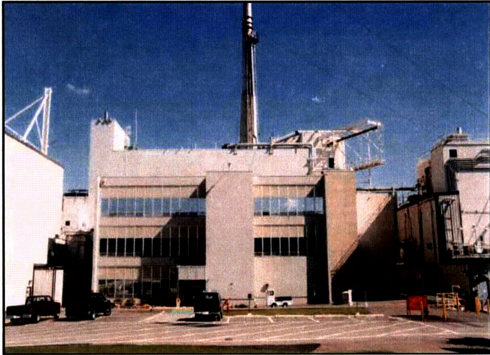
Figure 3-14. West Side of the Process Building. (The building with windows is actually the Plant Office Building. The plant part of the Process Building is behind the Office Building)
