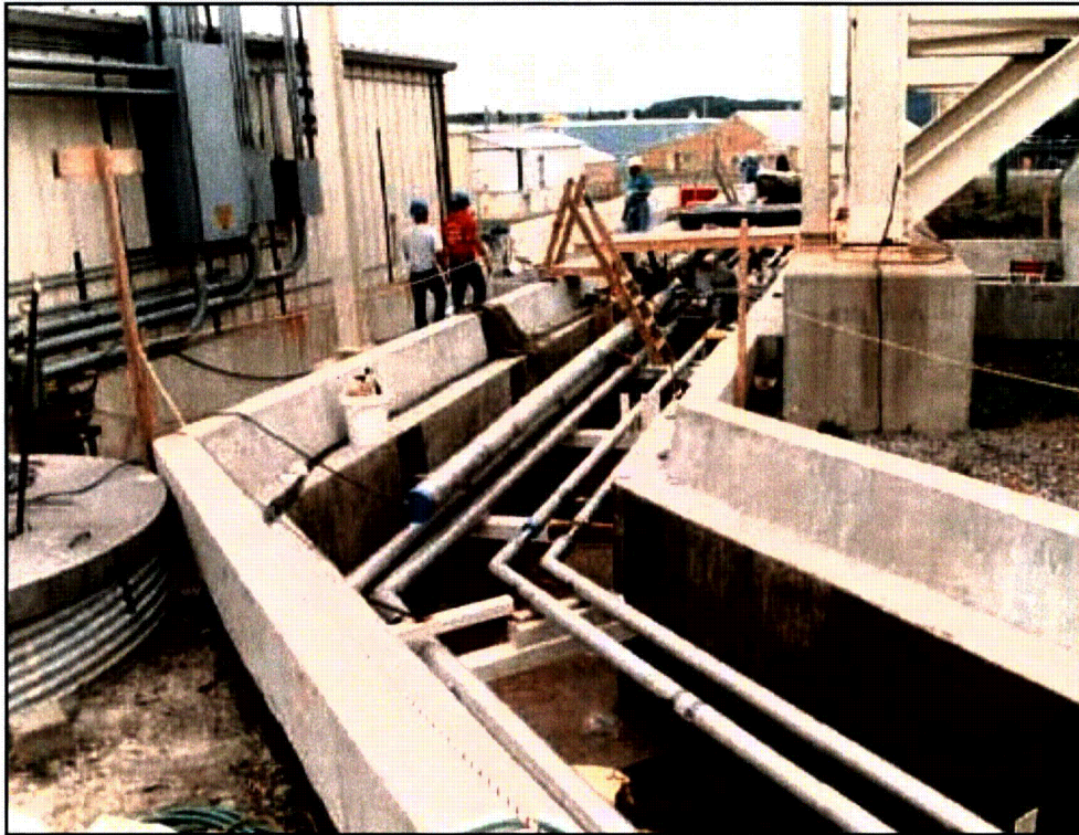
Figure 3-33. HLW Transfer Trench Under Construction
