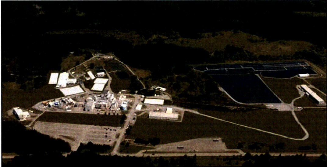
Figure 1-7. The WVDP in the Interim End State
