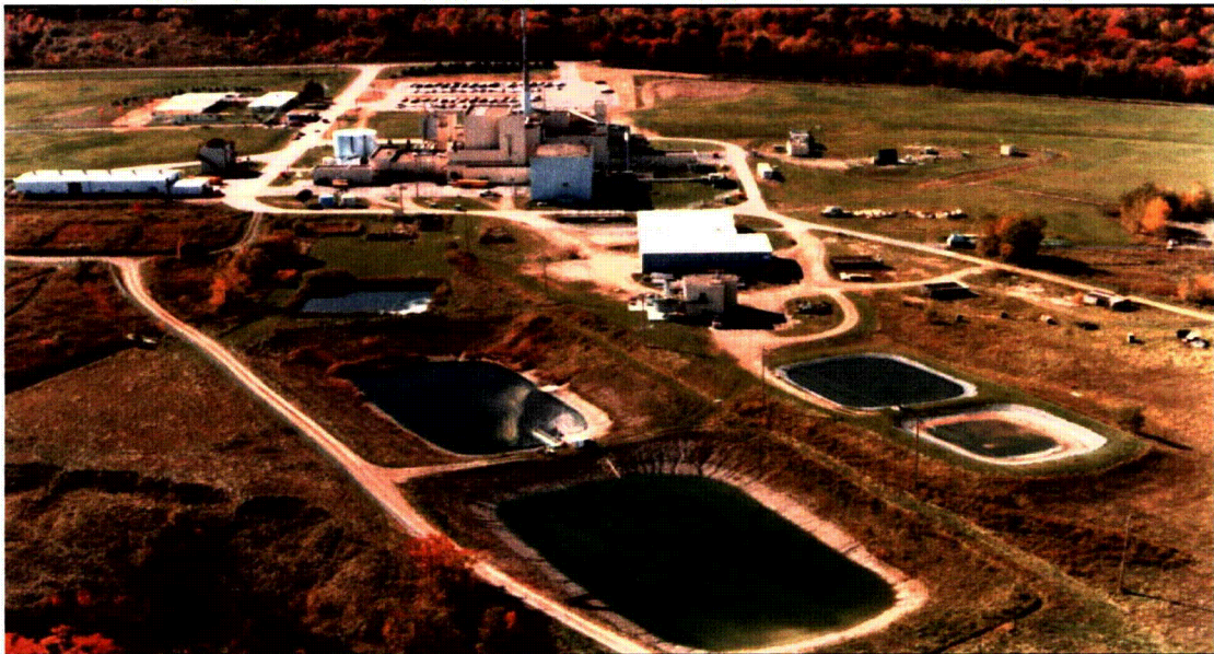
Figure ES-4. The Plant During the Early Years (The lagoons appear in the foreground. The Process Building can be seen in the background.)
