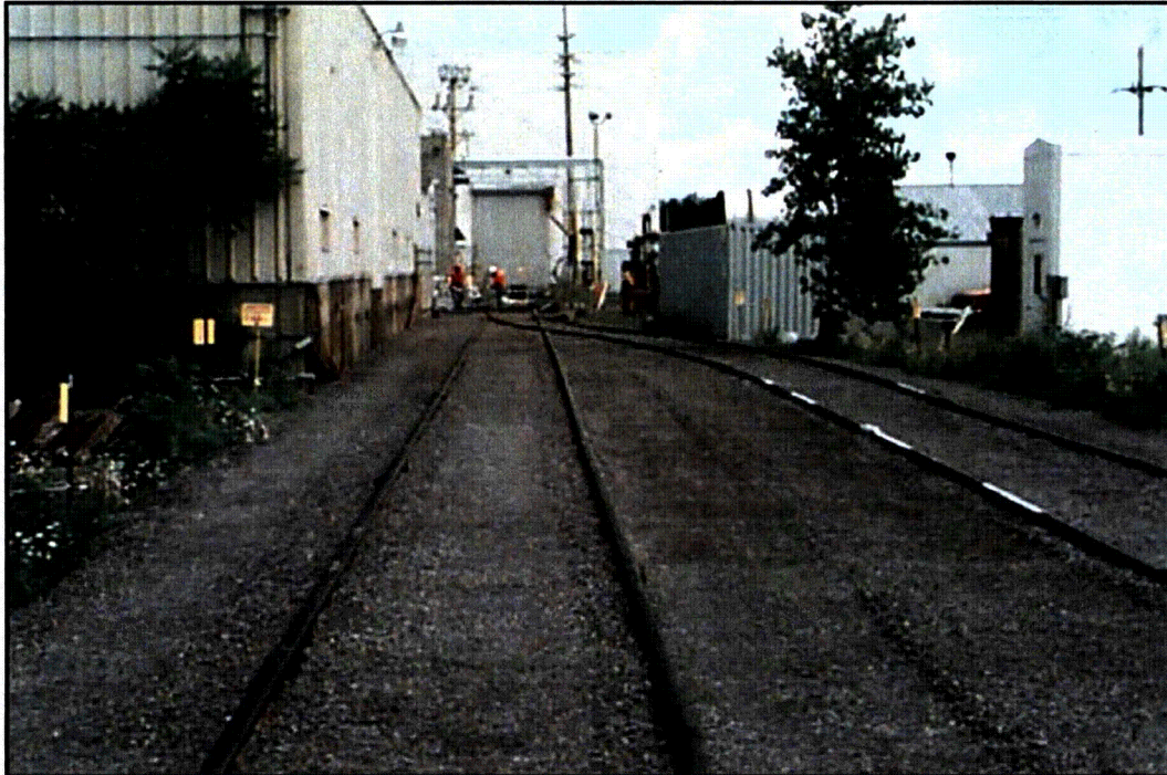
Figure 3-39. The Rail Spur. (The rail spur leads to the Fuel Receiving and Storage Facility.)
