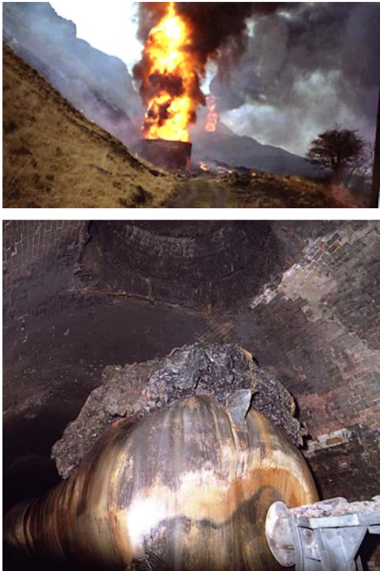
FIGURE 2.4 Photos from the December 1984 Summit Tunnel fire near Manchester, England. The top photo shows two fire plumes emerging from tunnel ventilation shafts. The bottom photo is an interior view of the tunnel. Part of the tunnel ceiling has collapsed onto one of the tank cars. SOURCE: Photos taken by a member of the West Yorkshire Fire Brigade or Manchester Fire Brigade (used with permission of www.todchat.com ).
