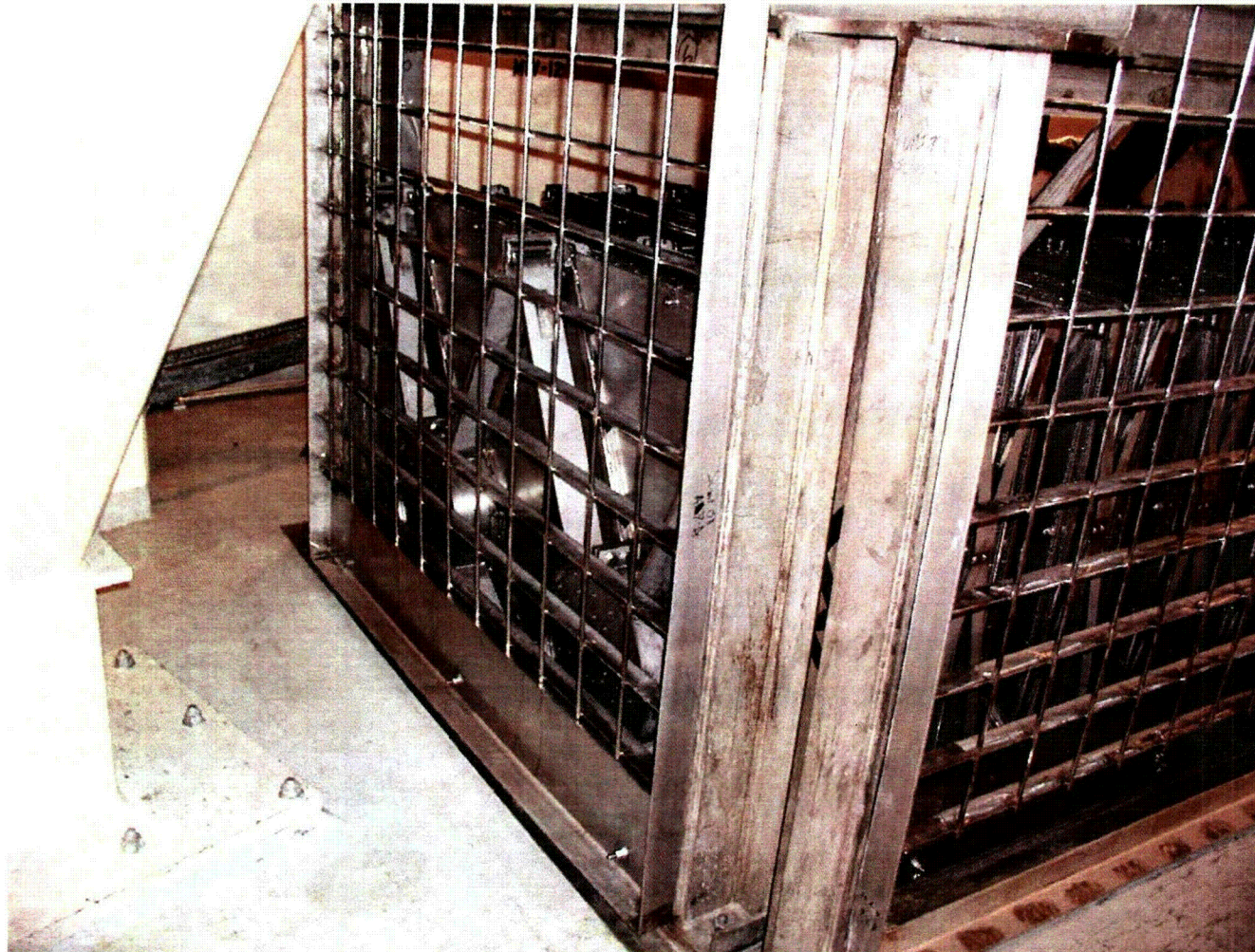
P-3.j.2-3 New Sump Strainer
