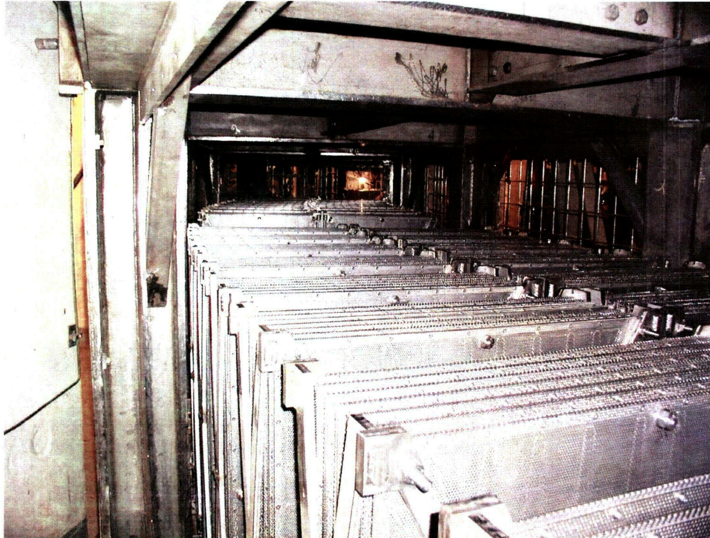
P-3.j.2-4 New Sump Strainer
