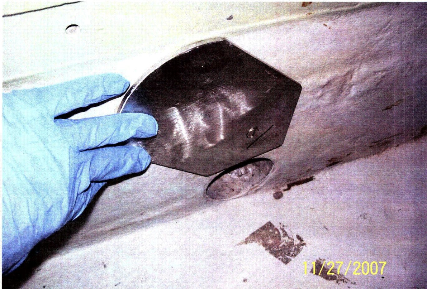
P-3.J.3-3 Normal sump drain cover
