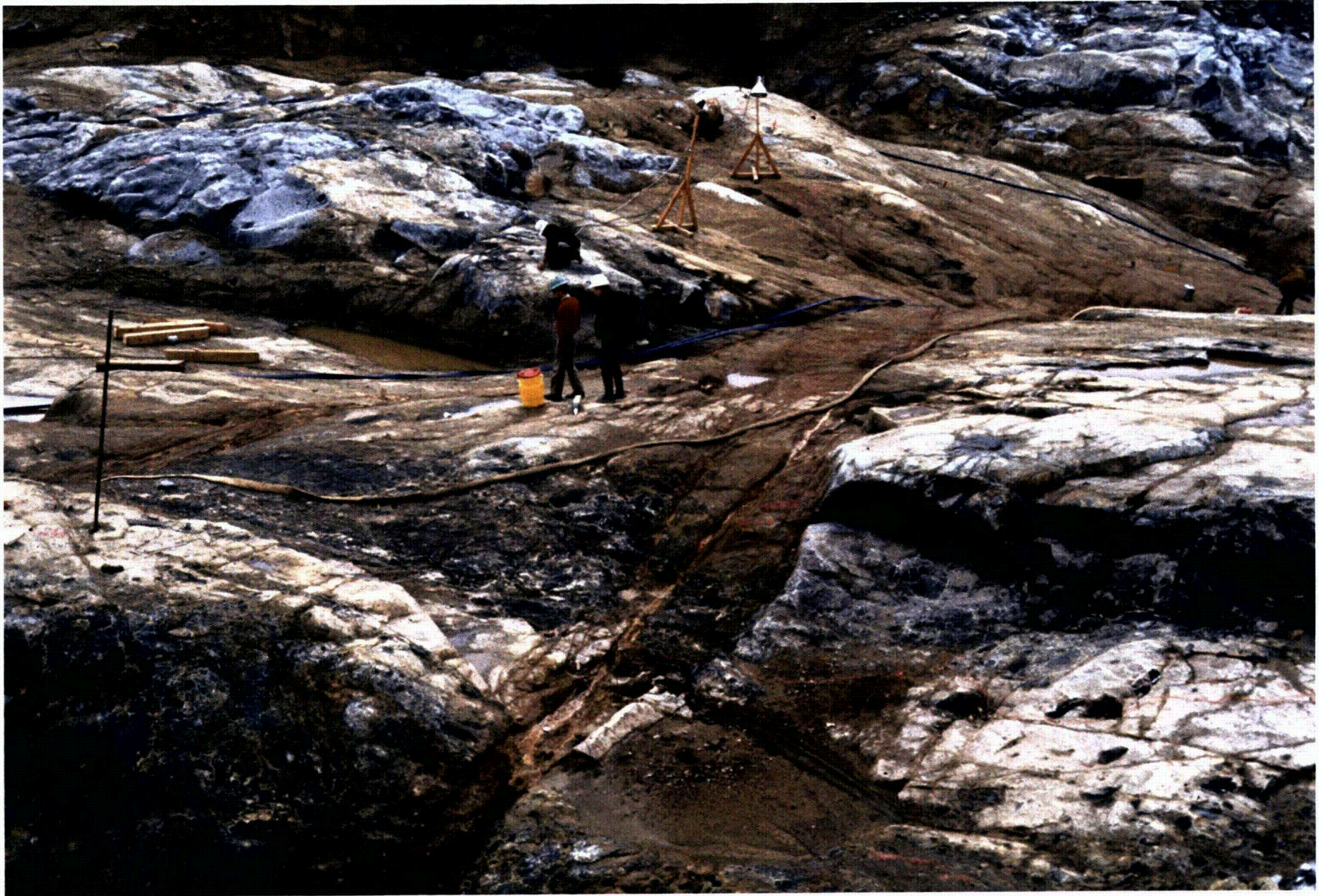
POWERBLOCK EXCAVATION TO BEDROCK – SOUTH VIEW (SHEAR FRACTURE RUNNING FROM NE/SW ACROSS CONTAINMENT BUILDING)
