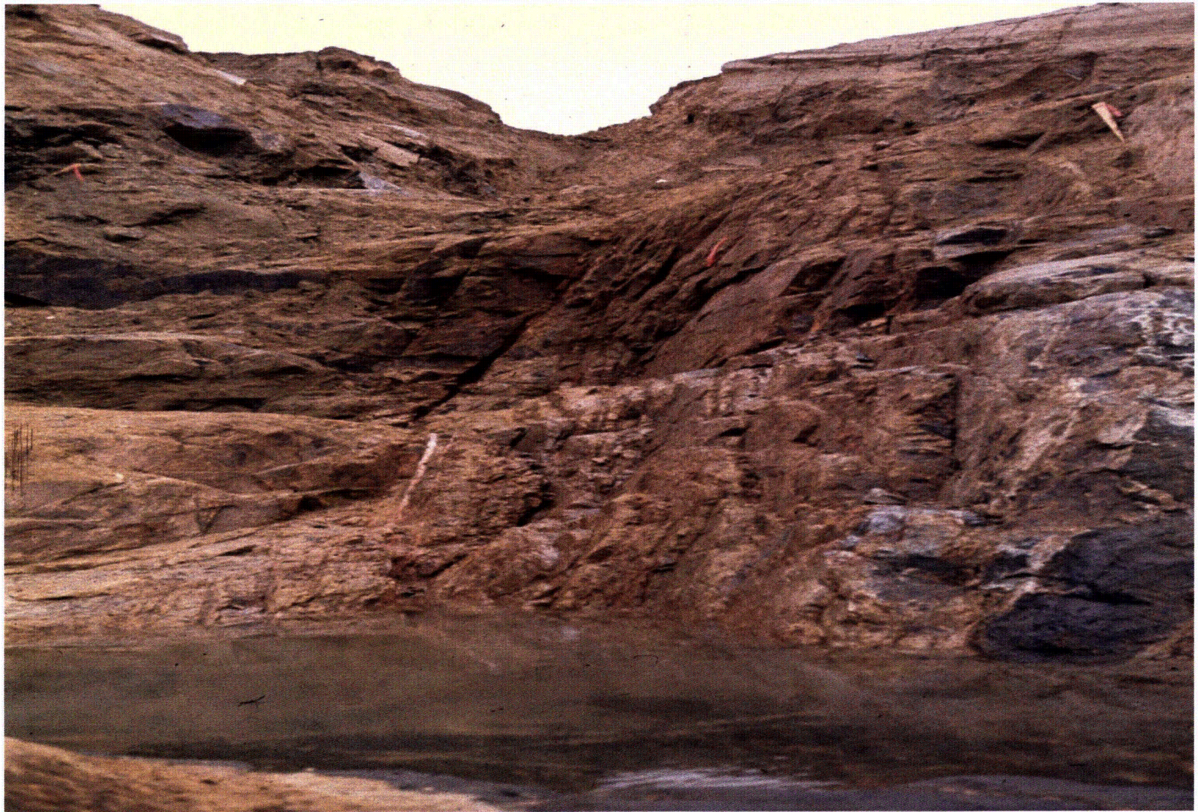
SIDE SLOPE OF POWERBLOCK EXCAVATION – TRANSITION OF ROCK TO SOILS
