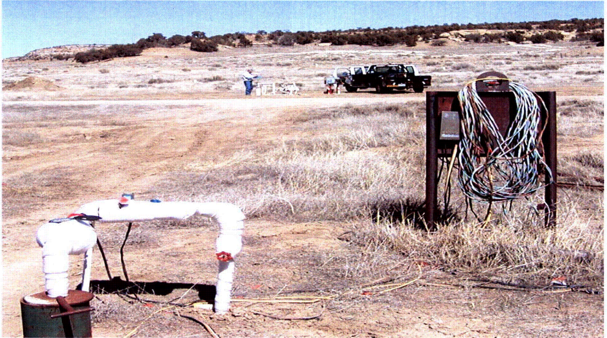
Photo 5. Zone 3 Well RW11 in foreground. Installed for hydrofracturing study; now an extraction well. Zone 3 monitoring wells in background. Well sampling ongoing in center background (looking north).
