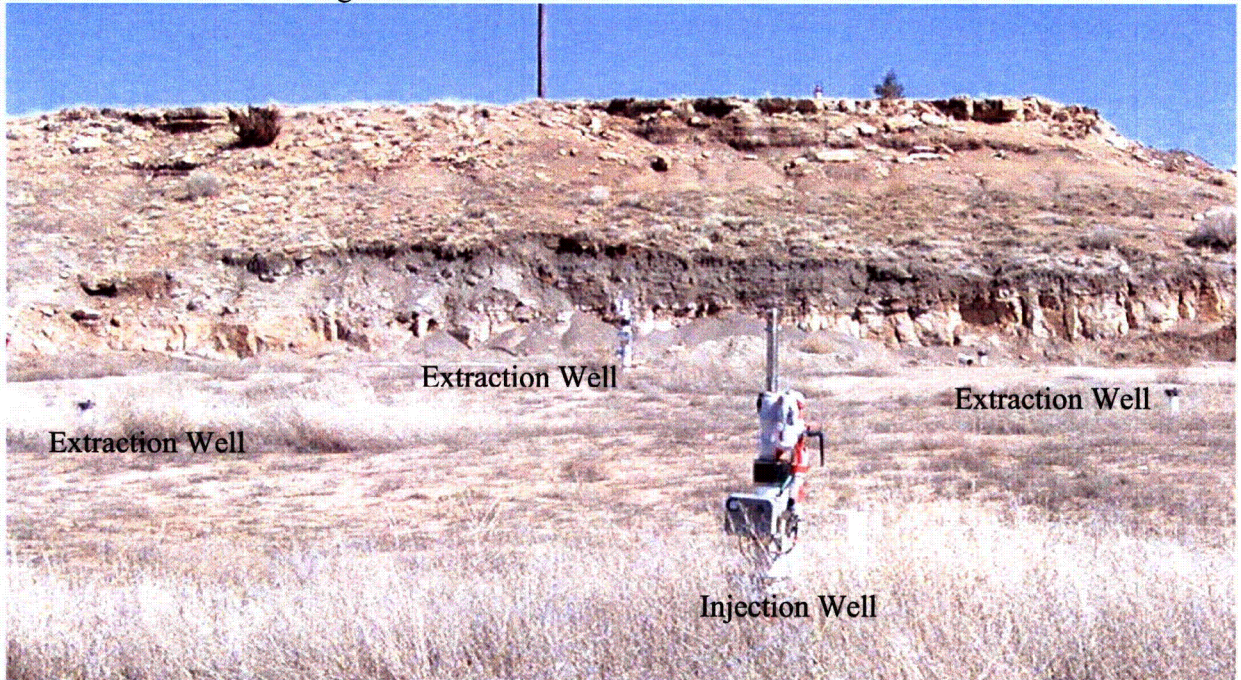
Photo 6. In Situ Alkalinity Stabilization Pilot Study site. Injection well in center; three extraction wells in middle ground.
