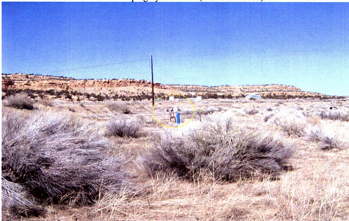
Photo 4. Southwest Alluvium Pumping System Well (shut off in 2001).
