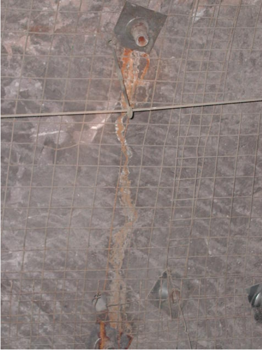
This photo was taken by Kevin Smart on April 18, 2006. The staining from the rock bolt down the side of the drift ceiling and wall are evidence that sufficient water drained down the rock bolt within the rock mass such that the resulting solute had enough mass and enough mineralization to stain a long pathway on the wall.
