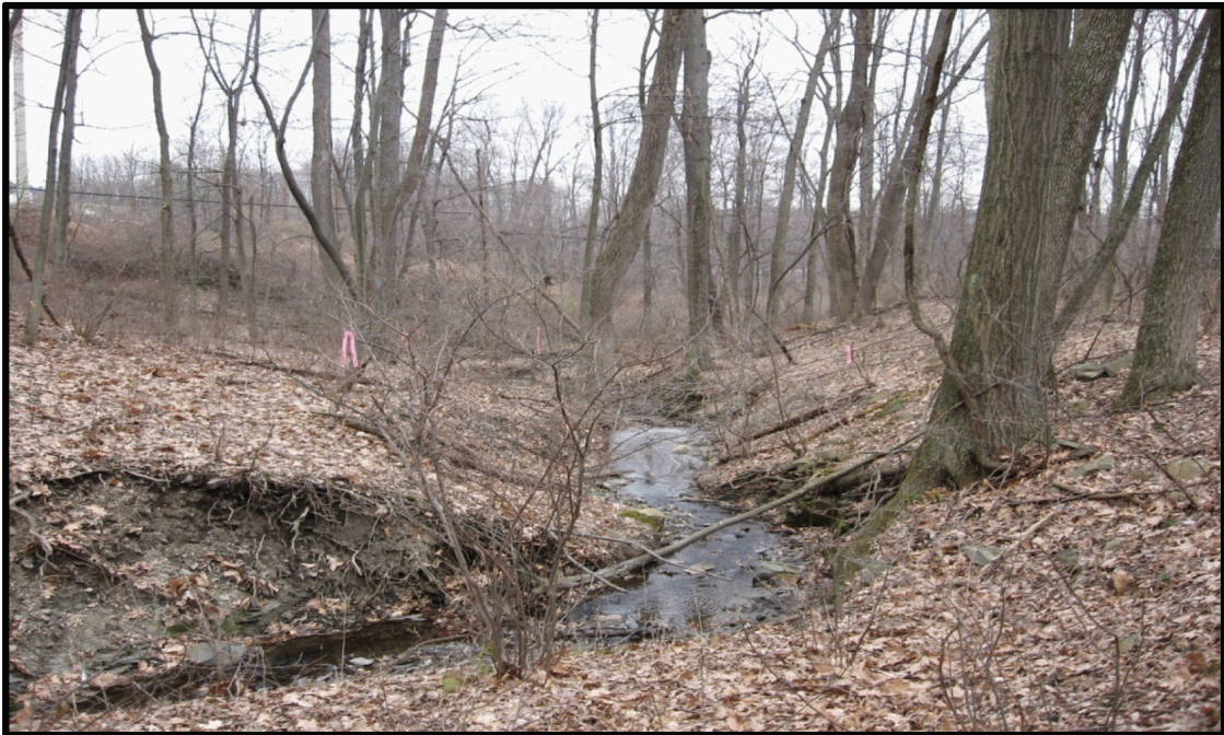
55. Scouring is common along the stream banks.
