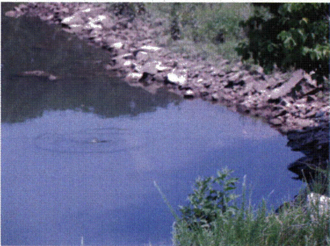
Figure 9: View of small whirlpool above inlet structure for 48" outlet pipe.
