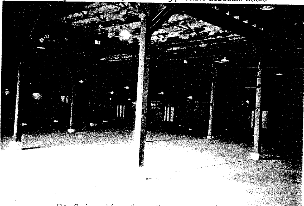
2 - Bay 2 viewed from the northwest corner of the bay
