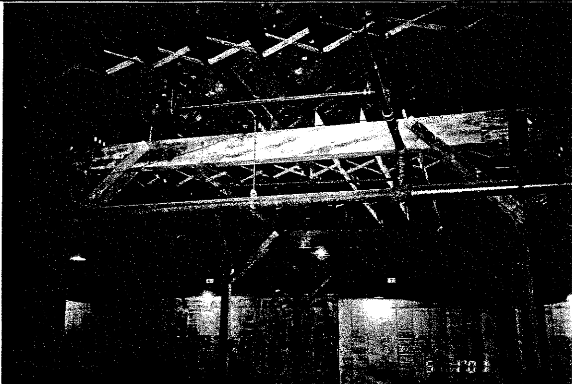
5 - Typical roof structure with fire sprinkler piping
