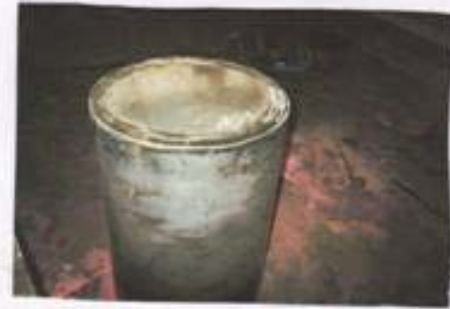
Completed Installation of Bottom Plug
