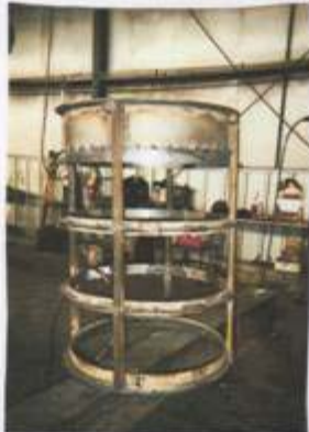
Skeleton of Secondary Containment Showing Reinforcement Rings and Vertical Stiffeners
