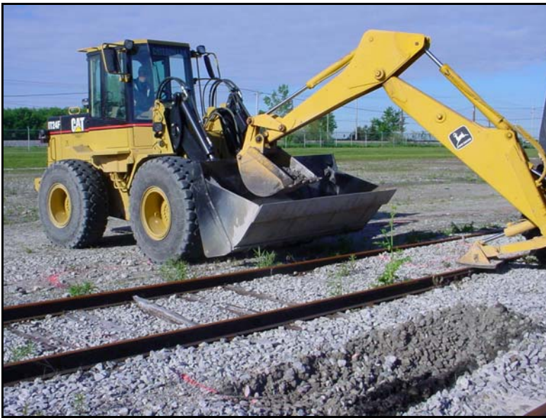
Transferring Material to Front-end Loader for Transport to 7A storage Cell
