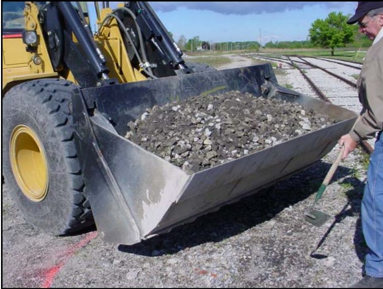
Maintaining the Material Below the Lip of the Bucket to Prevent Spillage During Transport
