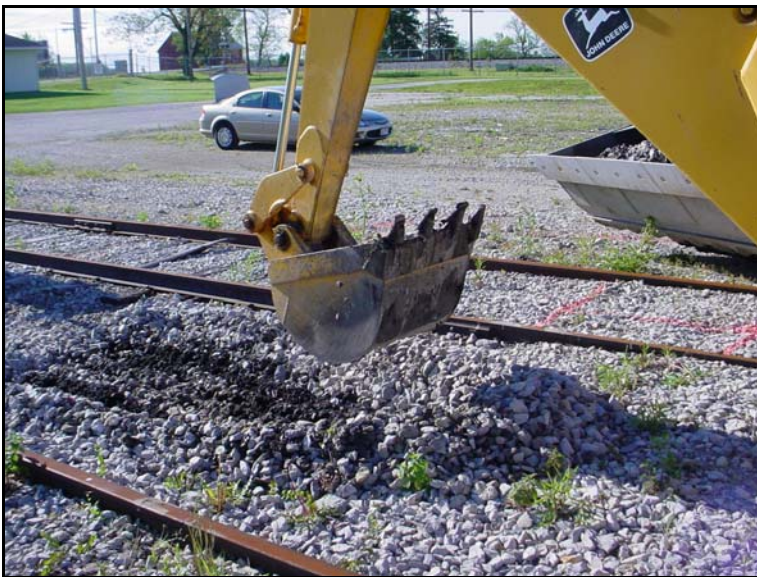
Removing Material Between North & South Tracks
