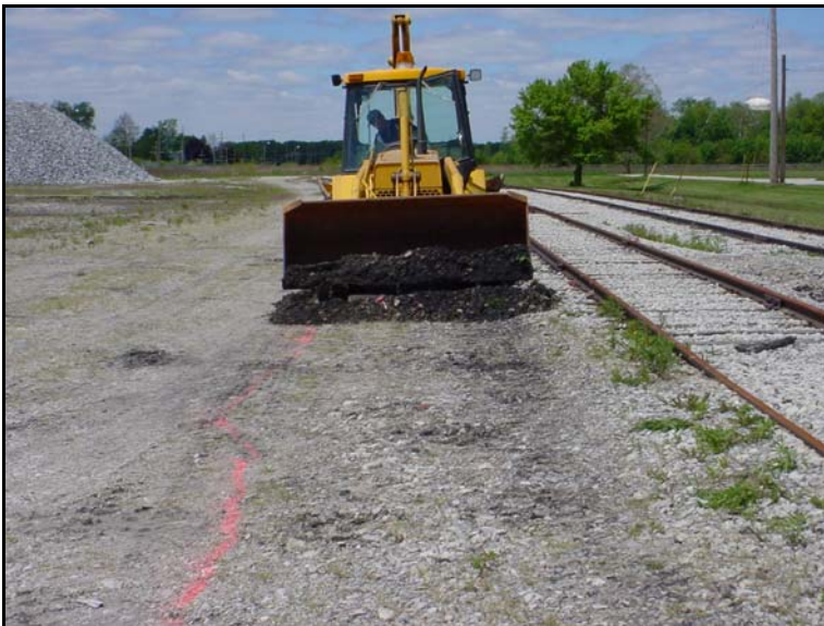
Scraping Material south of South Tracks
