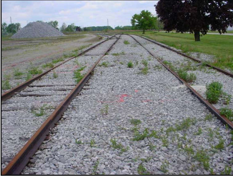
Area Between North & South Tracks to be Cleaned
