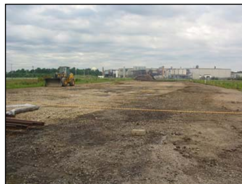
Figure 3. Darker areas of excavated area with elevated readings
