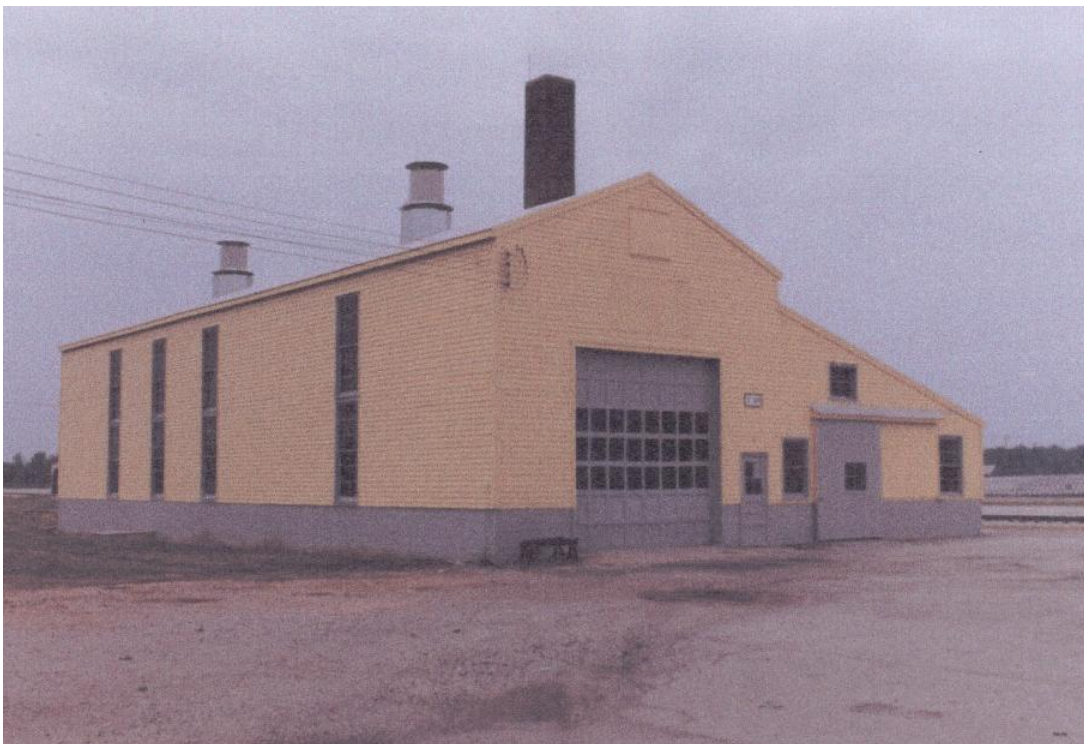
New Haven Depot, Building #124, Front View (circa 1981)
