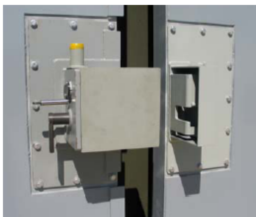
Figure 4. Internal Locking Device (ILD)
