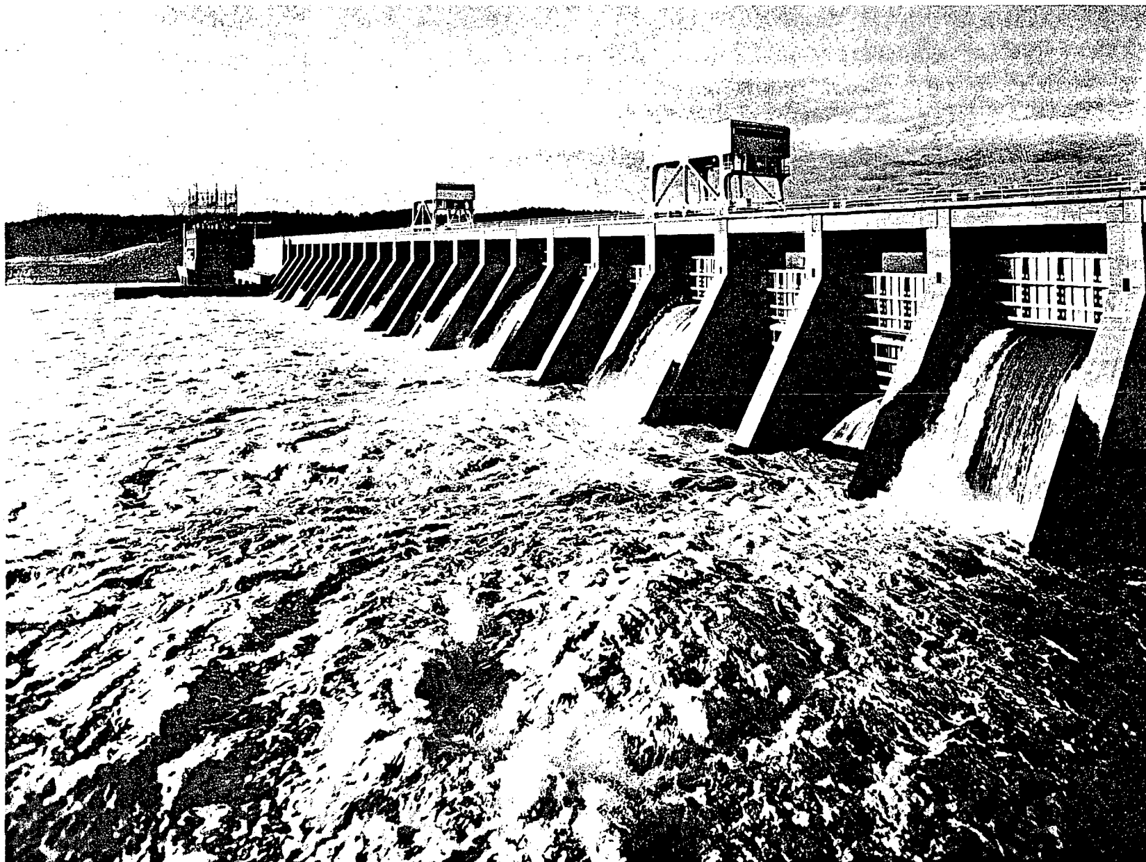
FIGURE 80.—Pickwick Landing Dam, a main river project, during a flood control operation.
