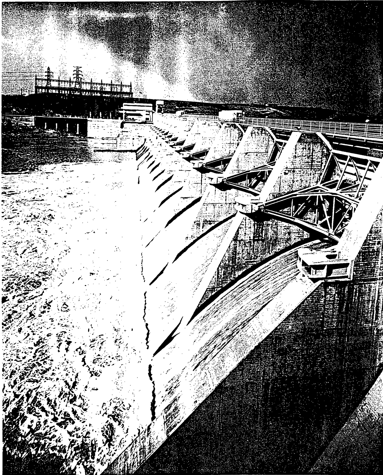
FIGURE 95.—Fort Loudoun Dam spilling water in excess of turbine requirements to bring reservoir to flood season level.
