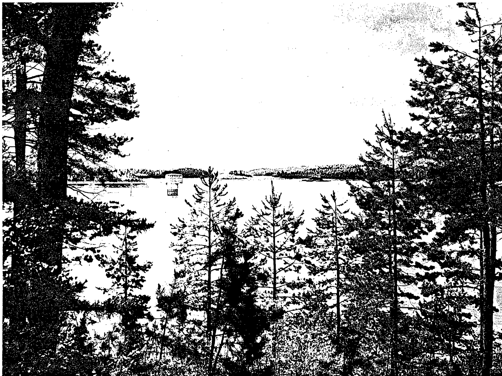
FIGURE 117.— Nottely Reservoir—stored floodwater reduces downstream flood elevations.
