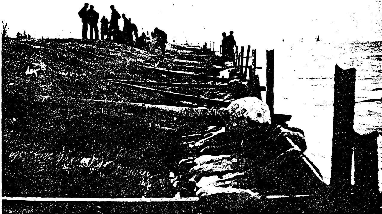
FIGURE 118.—Protecting Mississippi levee against wave wash during 1937 high water. (Large waves lashing the earth sides of the levees wash away the earth and are a serious menace to the levees. Here a crew of high water fighters has hastily constructed a board fence backed up by sand bags to protect the levee.)
