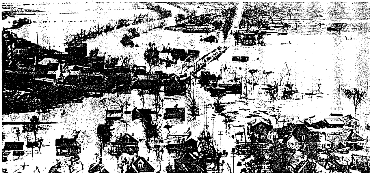
FIGURE 122.—Shelbyville during 1948 flood.
