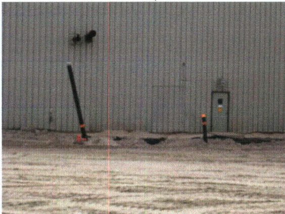
Seepage Collector #1 to the left
