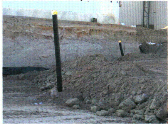
Seepage Collector #2 shown in background
