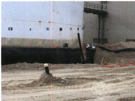
Seepage Collector #2 shown in background
