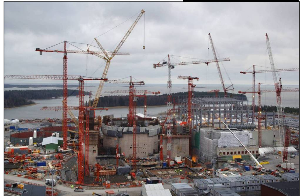
OL3 construction site
