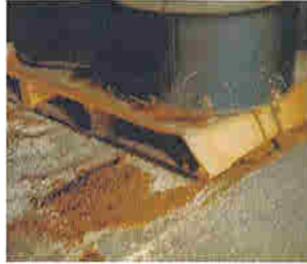
Figure 6 – Compromised Storage Drum
