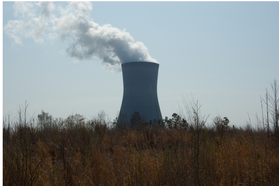
Harris Nuclear Power Plant
