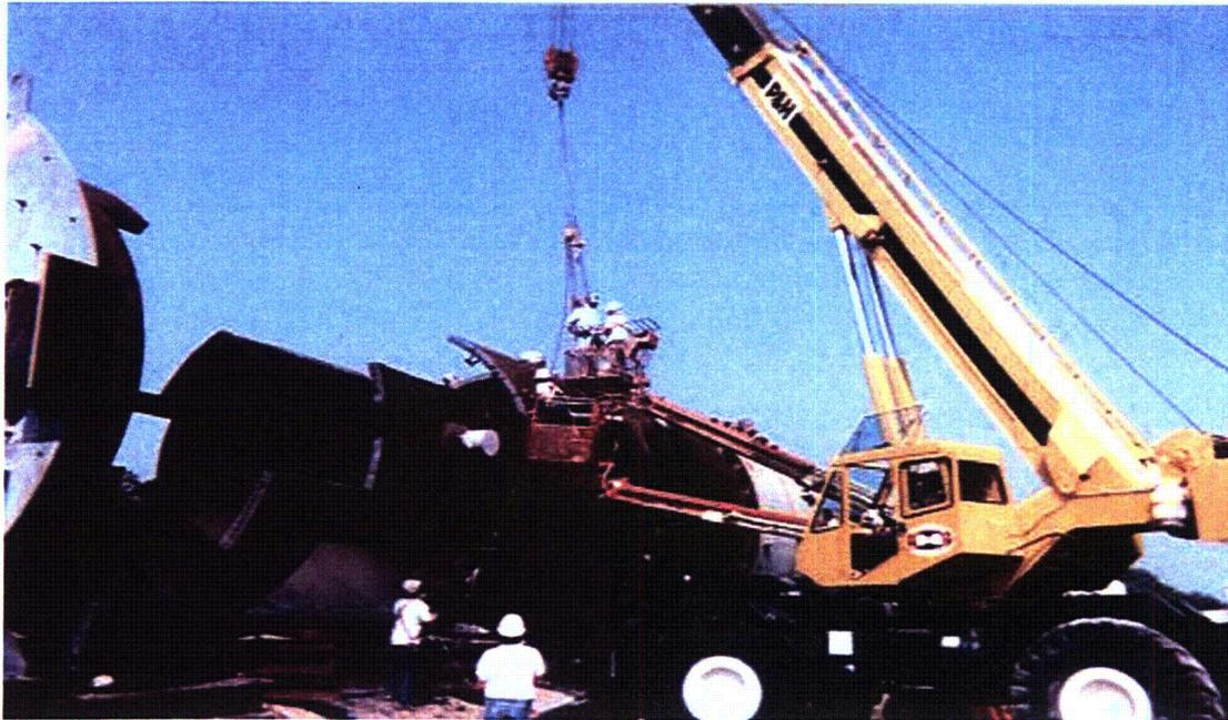
**Figure 3.9 River Bend Unit 2 RPV During Disassembly**
