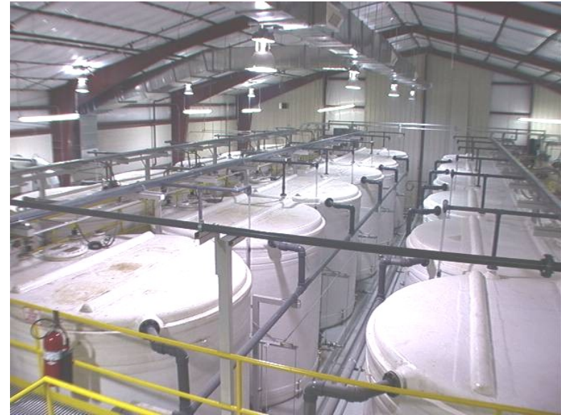
Uranyl Nitrate Building at NFS, Erwin, TN
