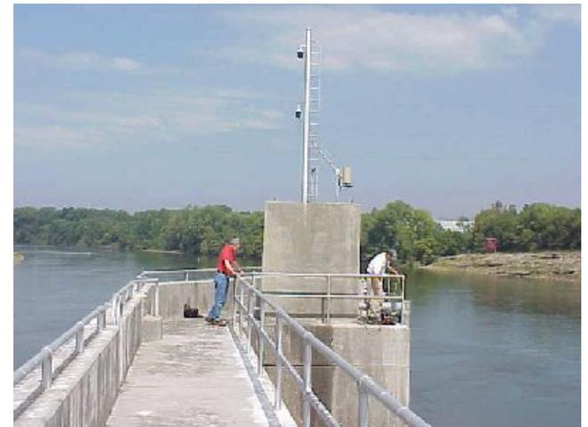
The water quality conditions in a deep pool can vary greatly with depth as the water column becomes stratified in response to seasonal temperature and flow patterns. During periods of stratification, water quality monitoring is conducted at several depths to evaluate effects of day-to-day operations.
