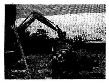
Metal debris is manually segregated from the screening line by the site worker. Also, the accompanying HP is scanning for changes in material activity as the line is operating. This is a continuous process. The picture is taken looking south across Section 2. Note that the picture was taken early July.
