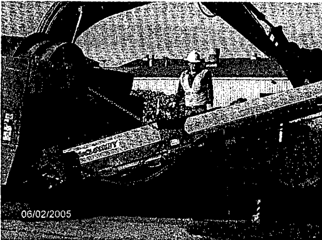
Figure 2. Material staged on the concrete pad, as potential LLRW, is further screened (2 nd iteration), to minimize LLRW volume.
