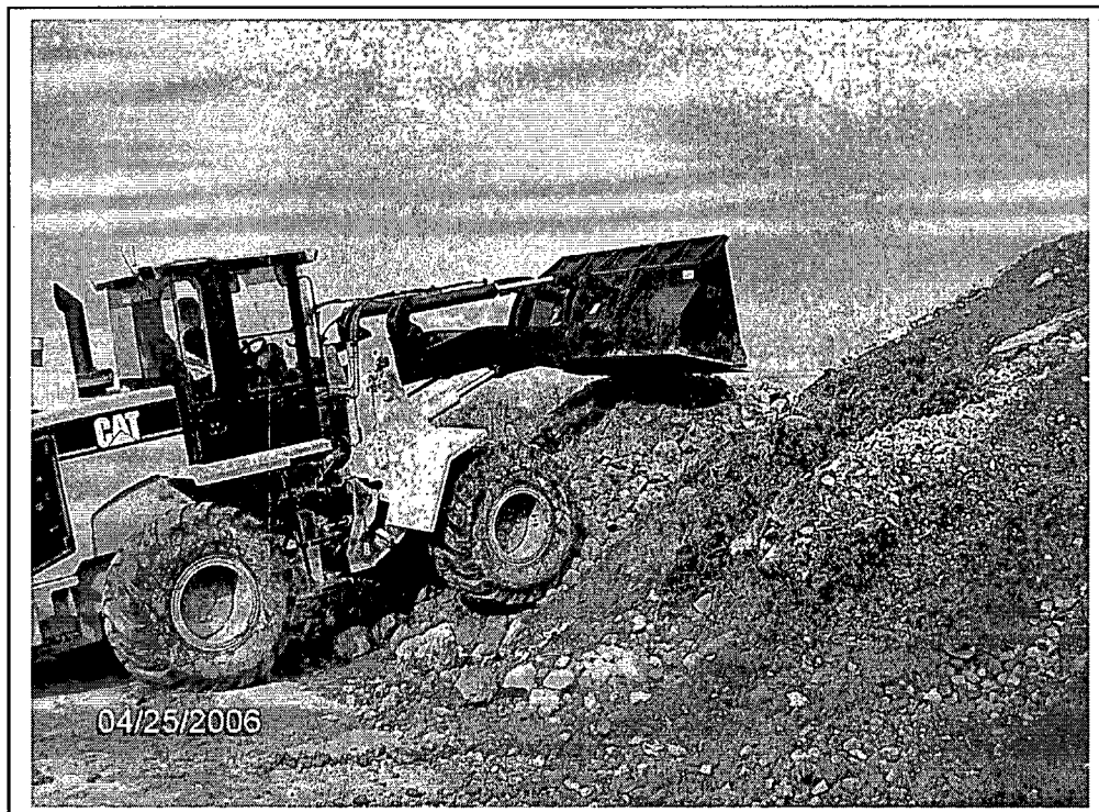
Waste pile is being prepared for loading on to trucks.
