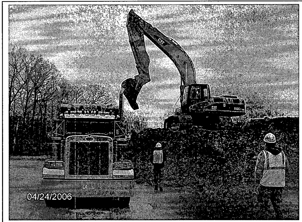
Day one of shipping waste staged on the pad begins. The schedule calls for fifteen truck loads a day carrying an average of 21.5 tons per truck.
