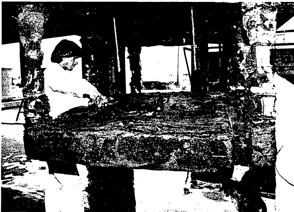
External stress skin removed from cable trays.
