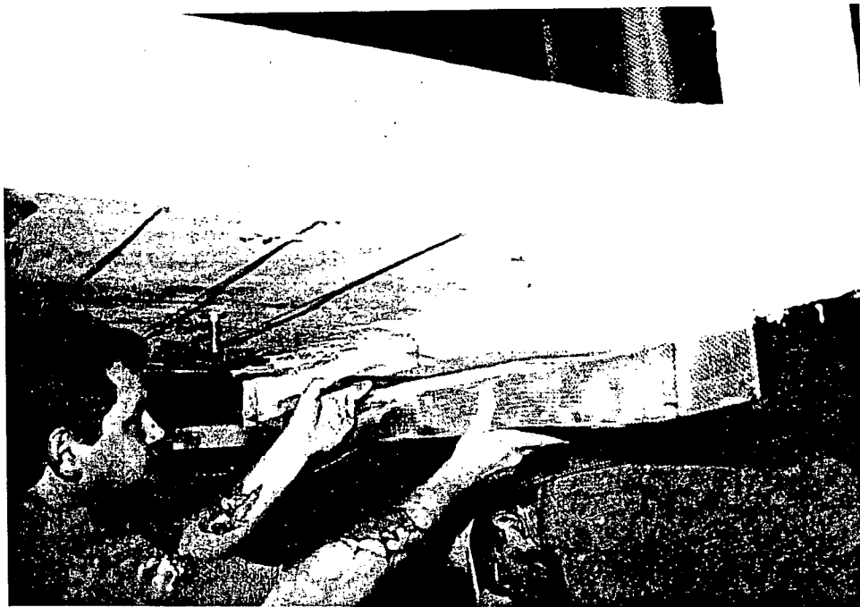
External stress skin fitted around horizontal support member.
