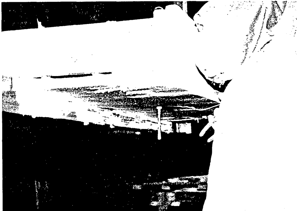
Panels held in place with washers and nuts and stainless steel tie wire.
