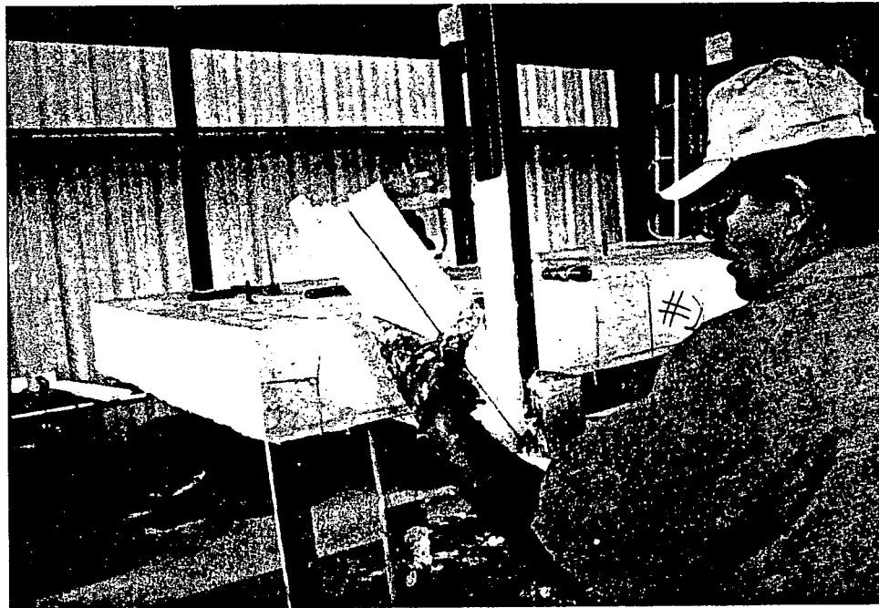
Pre-buttered panels installed onto support members.
