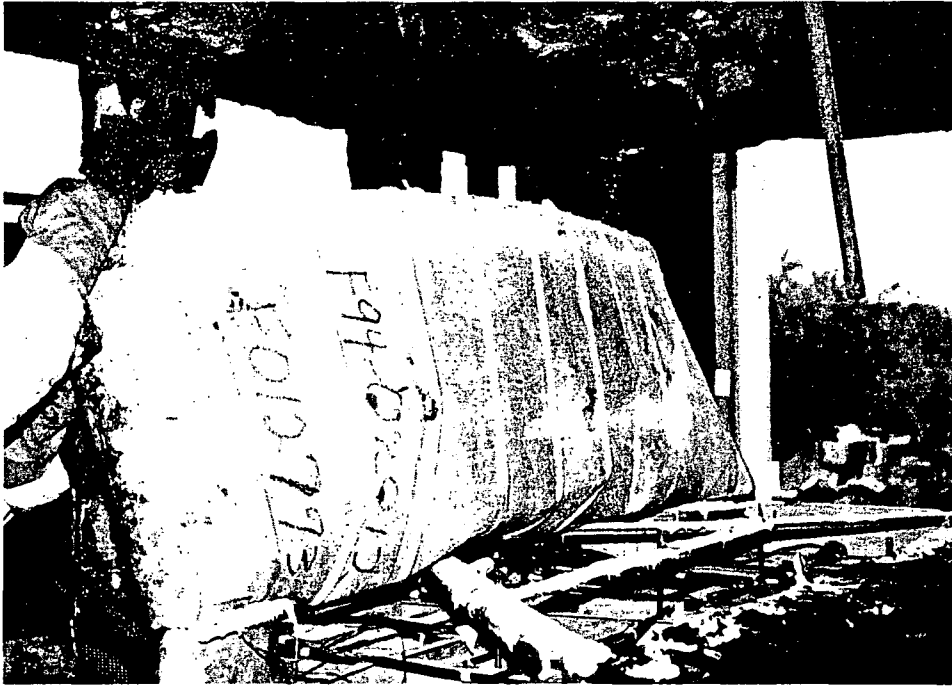
Material removed from top of fitting.
