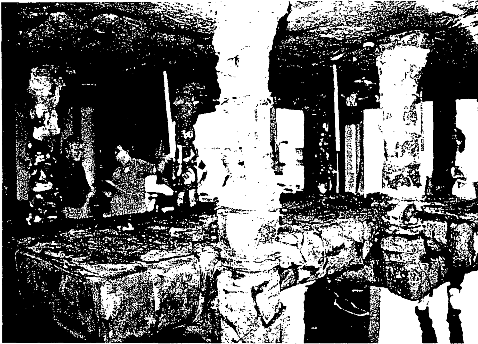
Rear of cable trays after hose stream test.
