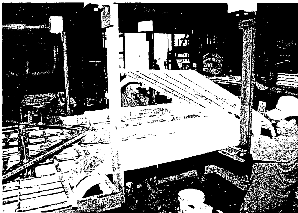
Pre-buttered panel installed on top of cable tray horizontal runs.
