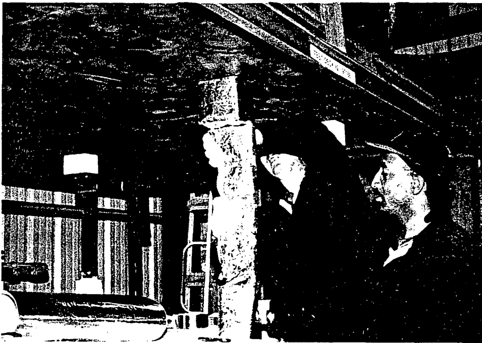
First layer of 3M material wrapped around vertical sections of support members.
