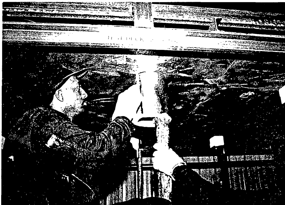
Second and final layer of 3M material installed on top of support member.
