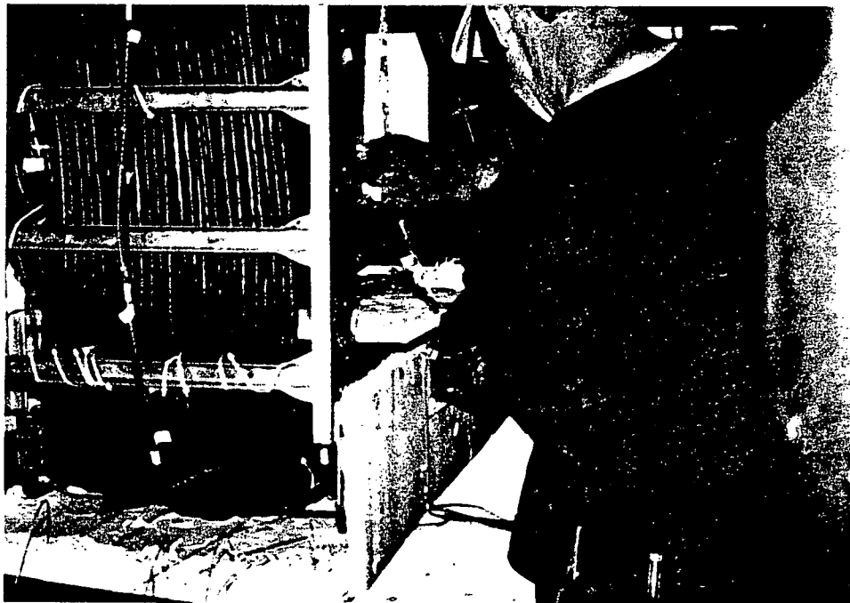
Cables installed into 5 in. air drop.
