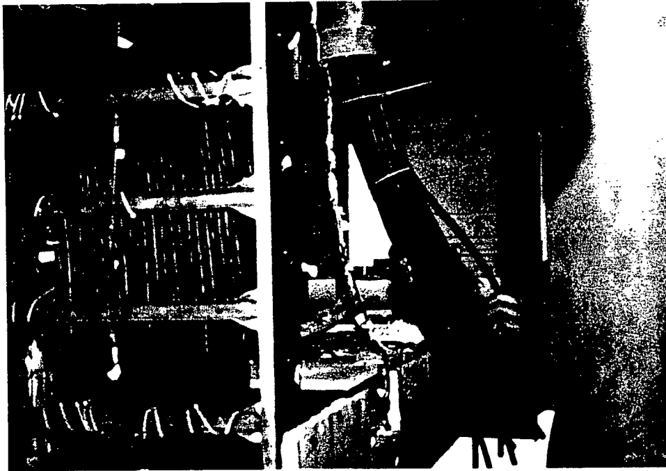
Cables installed into 5 in. air drop.
