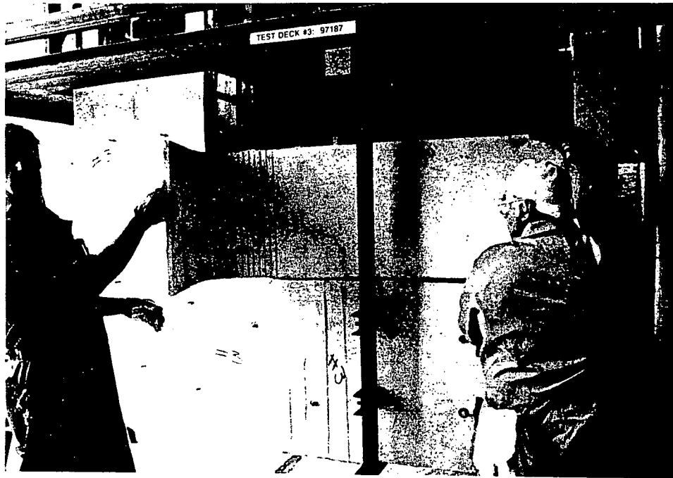
Scored and folded panel installed on top of common enclosure portion of trays.
