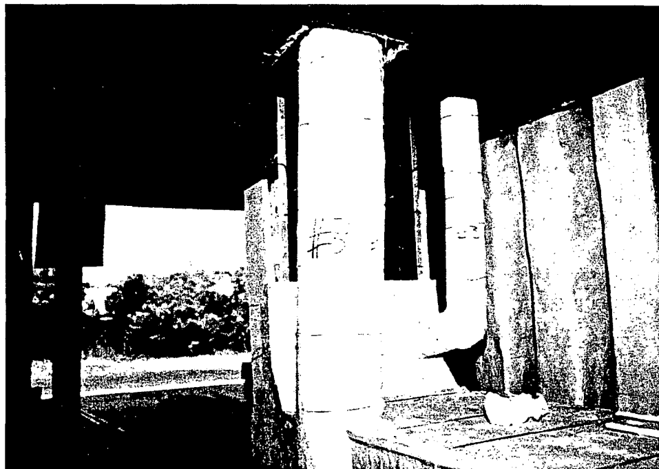
Overlay of pre-shaped conduit sections installed on 1 in. air drop.
