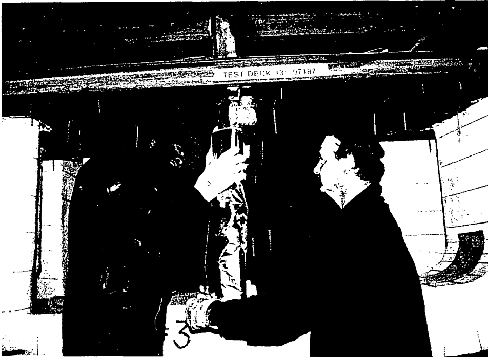
First layer of 3M material installed on support members.
