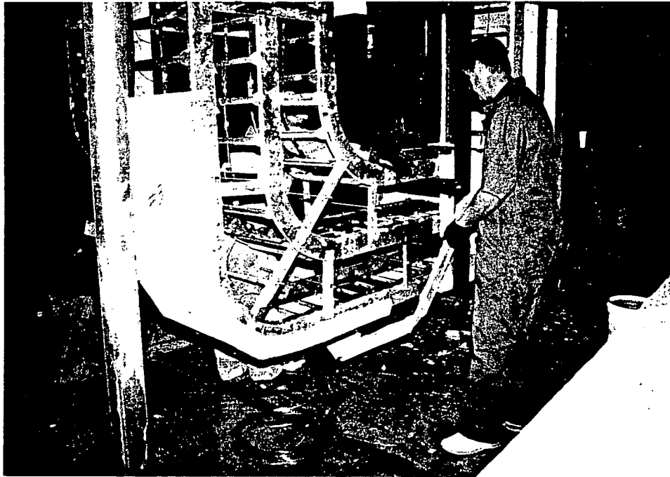
Scored and folded panel installed in common enclosure portion of trays.
