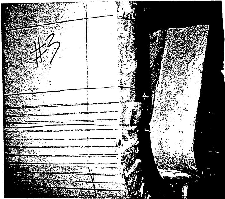
Pre-buttered, scored and folded panel installed on inside of rear tray radial bend.
