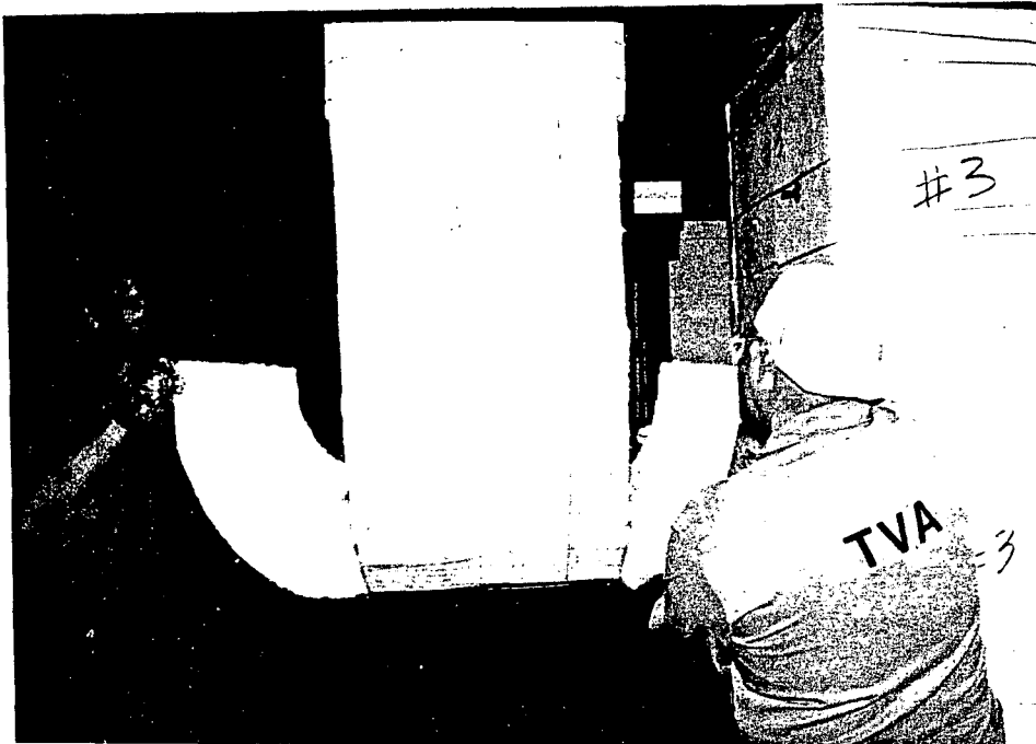
Pre-buttered panels installed on sides of radial bend on rear tray.
