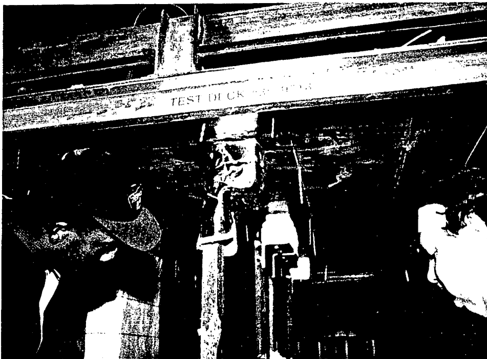
3M material installed on tops of support members.
