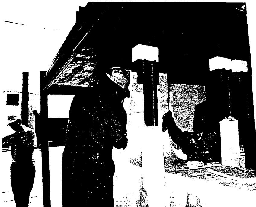
External stress skin overlay stapled into place on trays.
