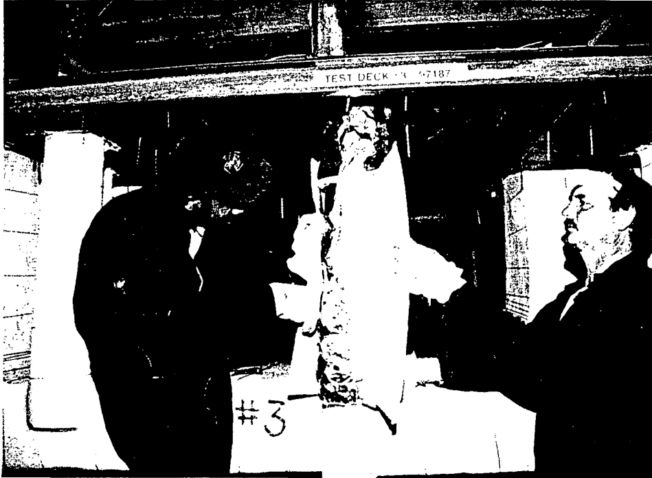
Third and final layer of 3M material installed on supports.
