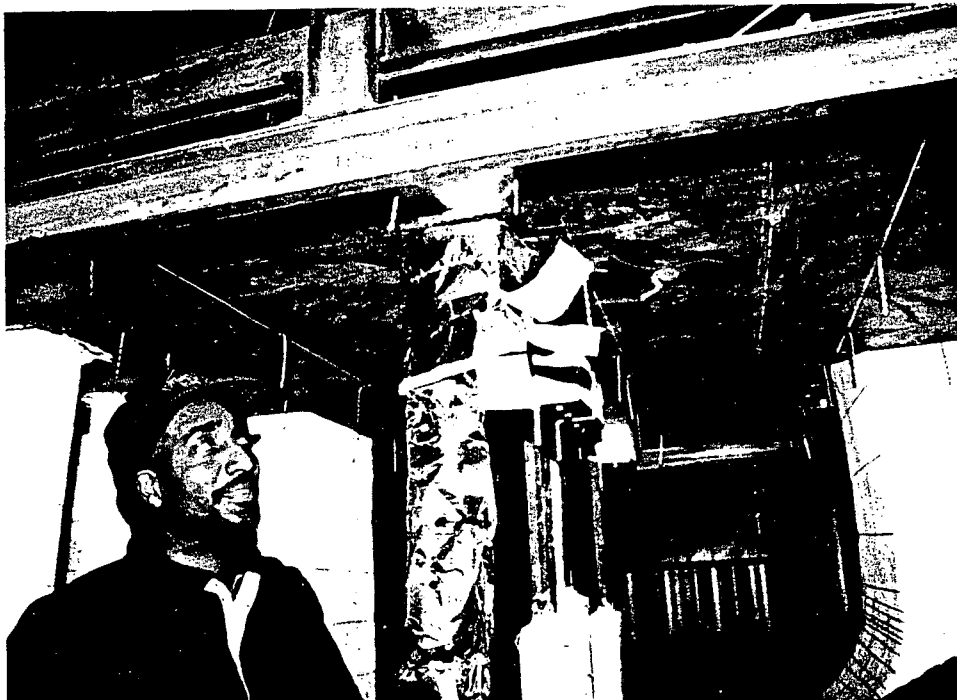
Second layer of 3M material installed on tops of support members.
