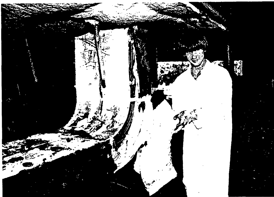
Material removed from side of rear tray radial bend.
