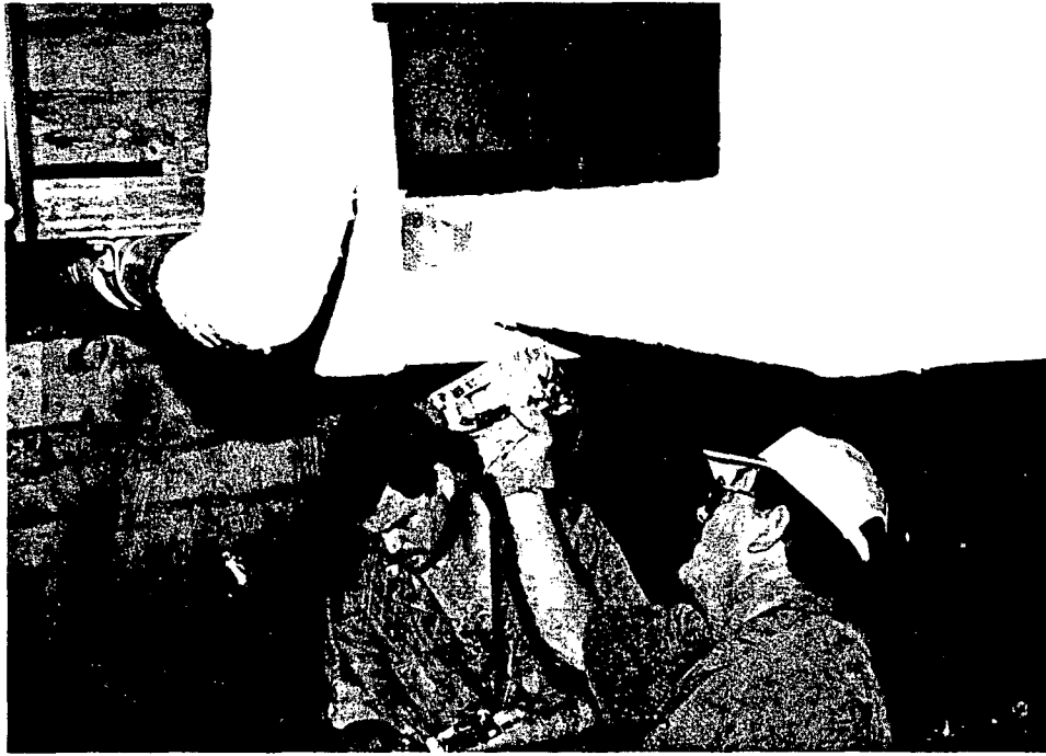
External stress skin secured to enclosures with staples.
