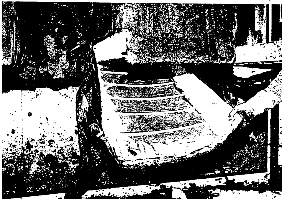
Material removed from bottom horizontal section of center cable tray.
