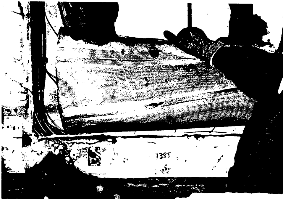
Material removed from top horizontal section of left cable tray.
