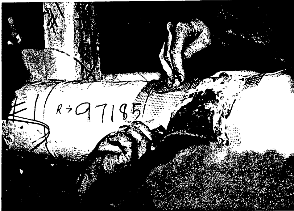
External stress skin wrap installed at joints in conduit run.
