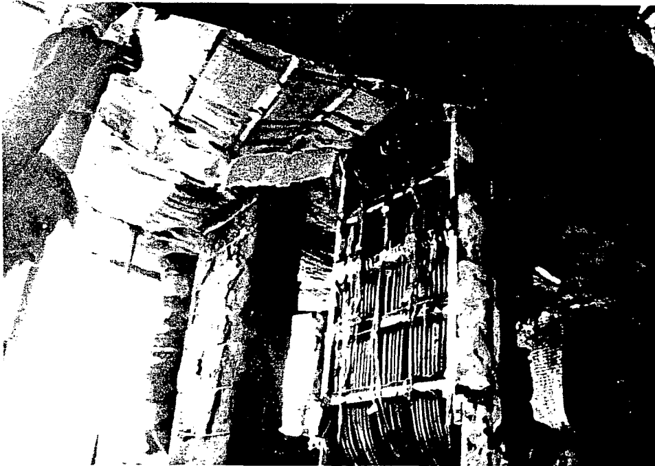
Cables in vertical section of center cable tray.
