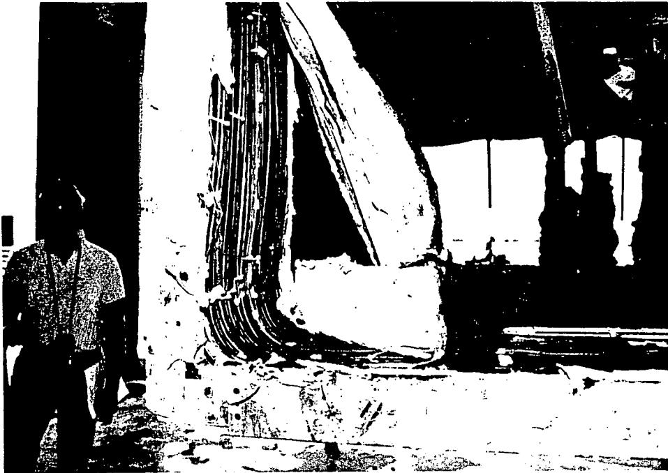
Cable in vertical and bend area sections of left cable tray.
