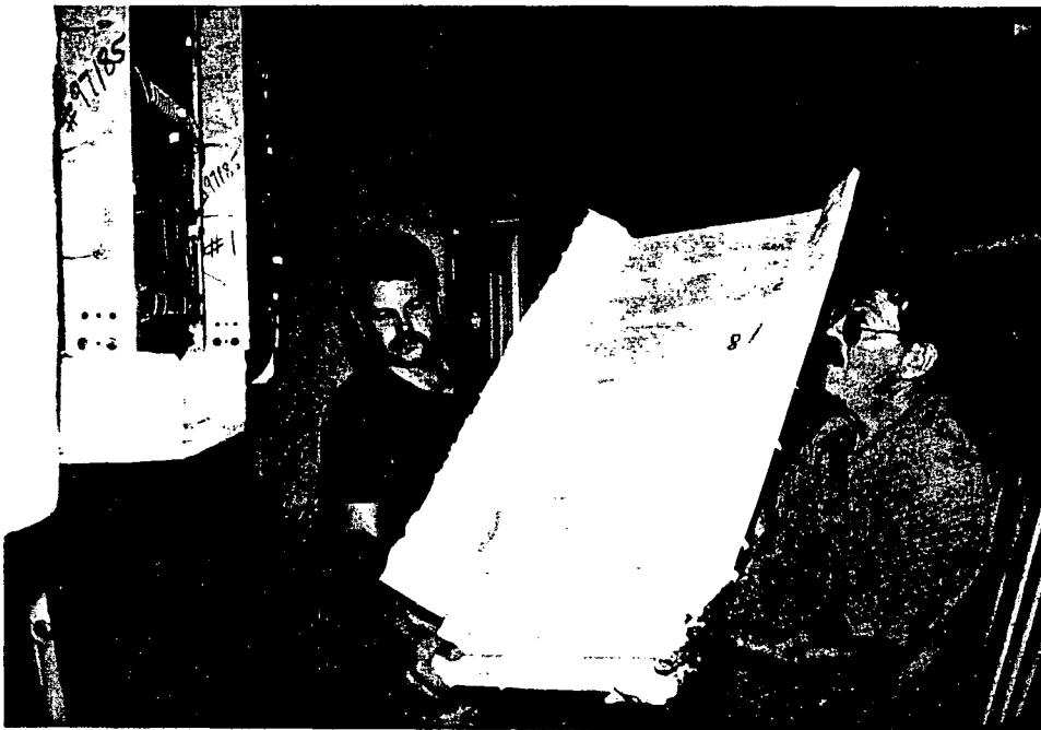
Pre-buttered scored and folded panels installed onto outside vertical section.
