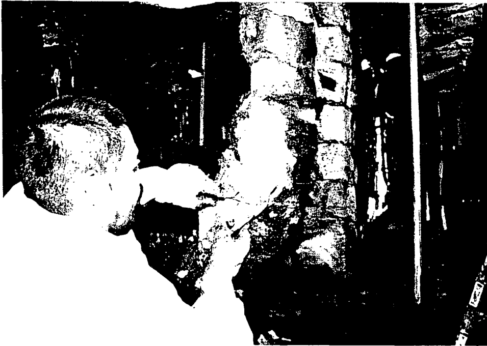
Material removed from radial section of conduit.
