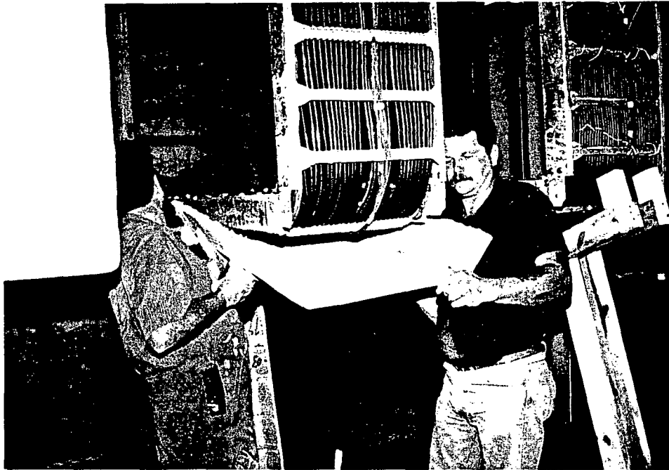
Pre-buttered scored and folded panels installed onto tray bottom and sides.
