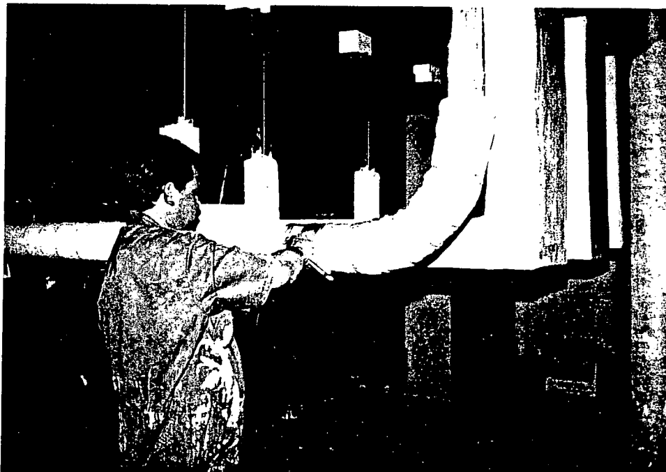
External stress skin wrap installed over conduit radial bend.
