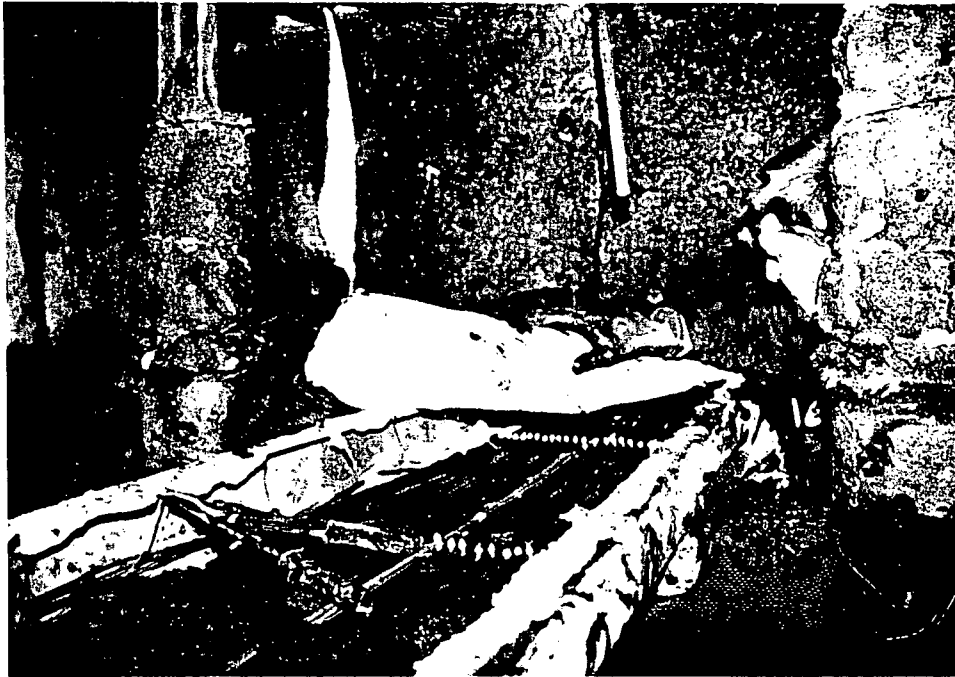
Material removed from horizontal section of center cable tray.
