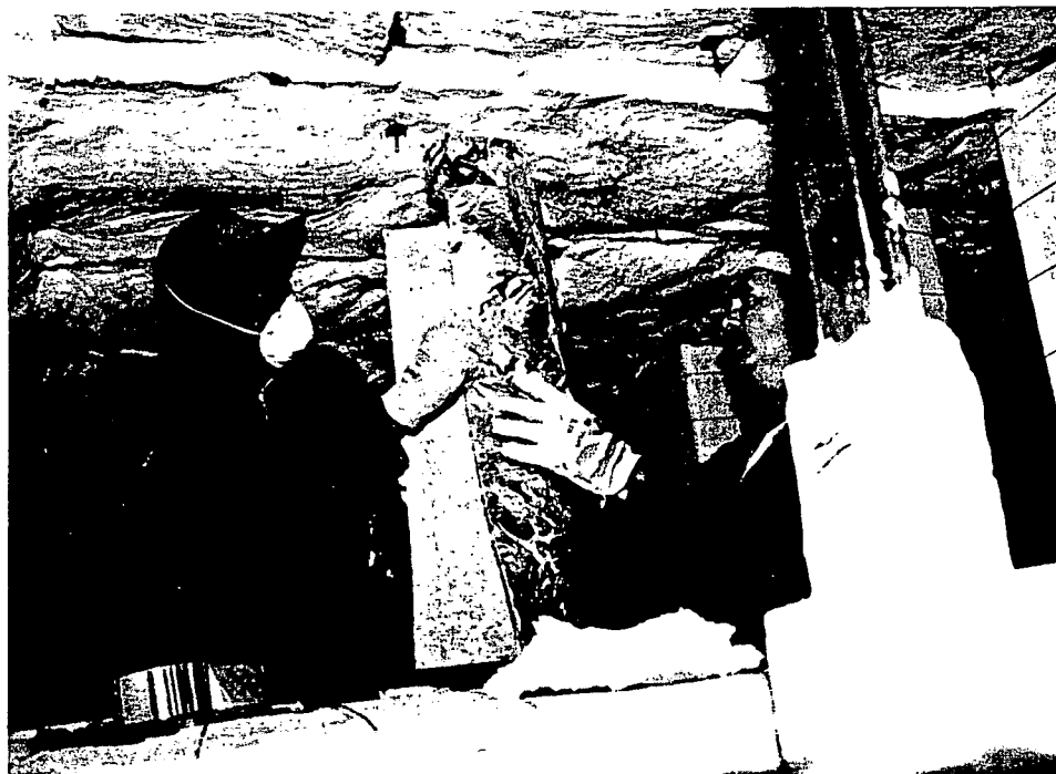
Single layer of 3M material wrapped around vertical support members.
