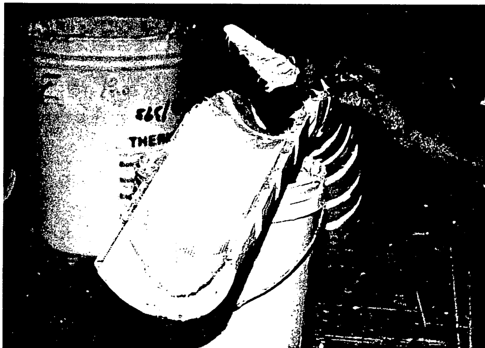
Bent pre-shaped conduit section pre-buttered prior to installation.
