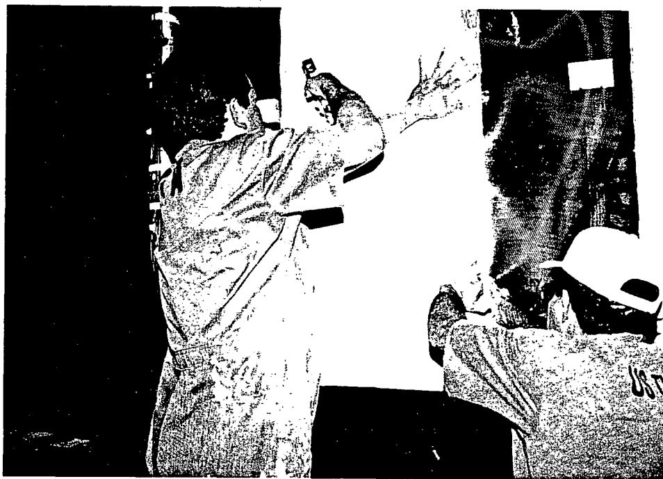
External stress skin stapled to vertical tray section.
