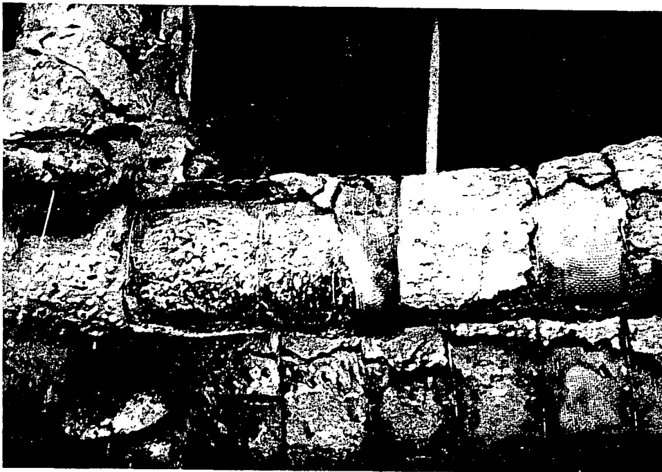
End of conduit radial bend section.
