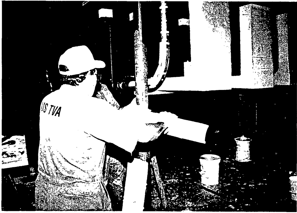
Notched pre-shaped conduit section bent into rough shape.
