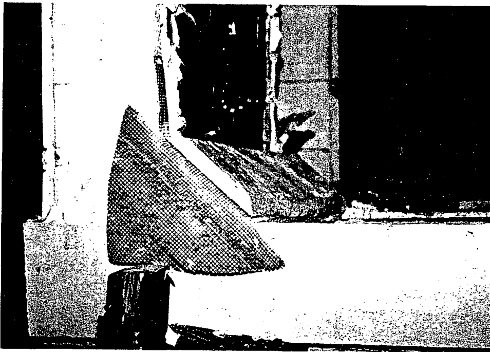
Section of panel installed over raised cables in bend area.
