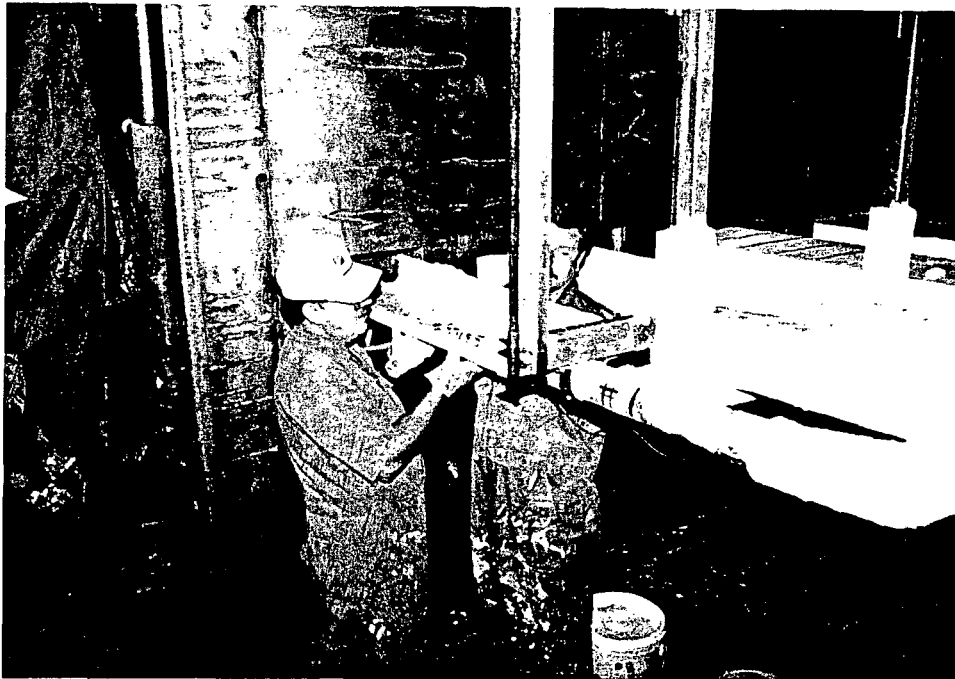
Pre-Buttered, pre-shaped conduit sections installed onto conduit horizontal run.
