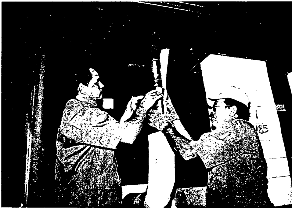
Material secured with foil tape.
