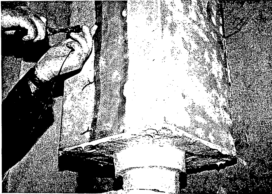
Joint in external stress skin stitched with stainless steel tie wire.
