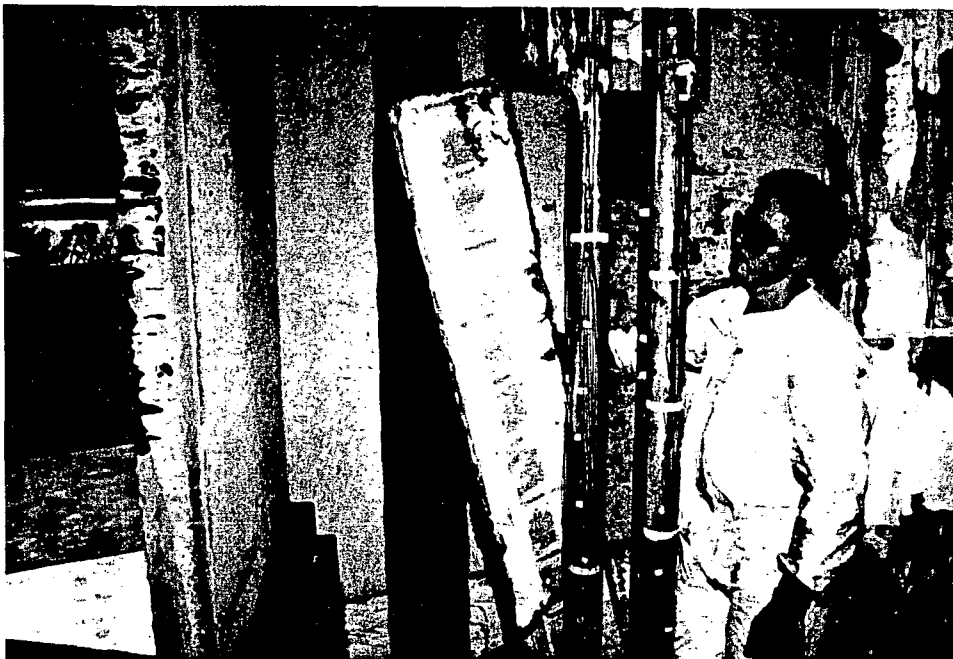
Material removed from lower rear of 3 in. enclosure.
