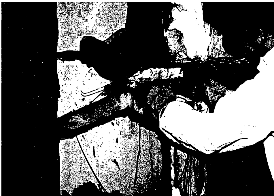
Material removed from support member below junction box.
