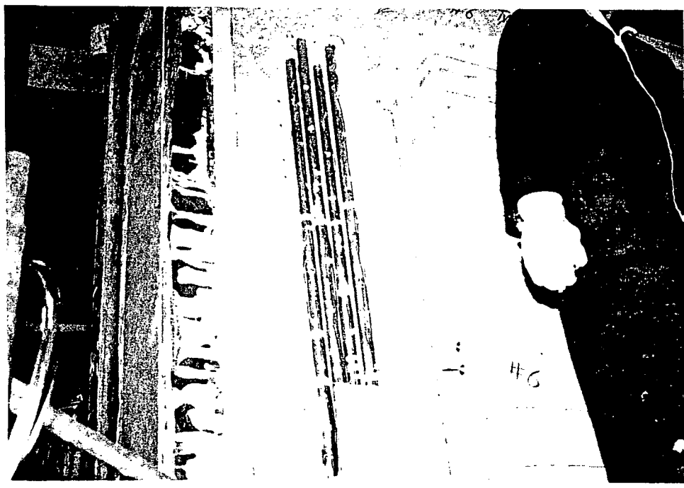
Upper base plate installed and panels in place on 3 in. conduit set.
