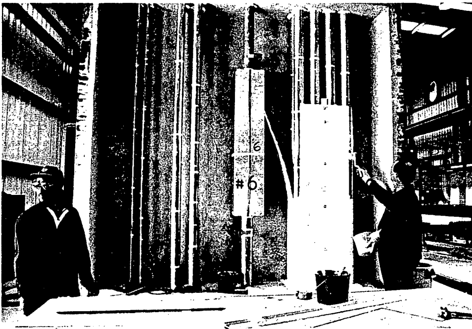
Sides of conduits and radial bends pre-buttered prior to panel installation.
