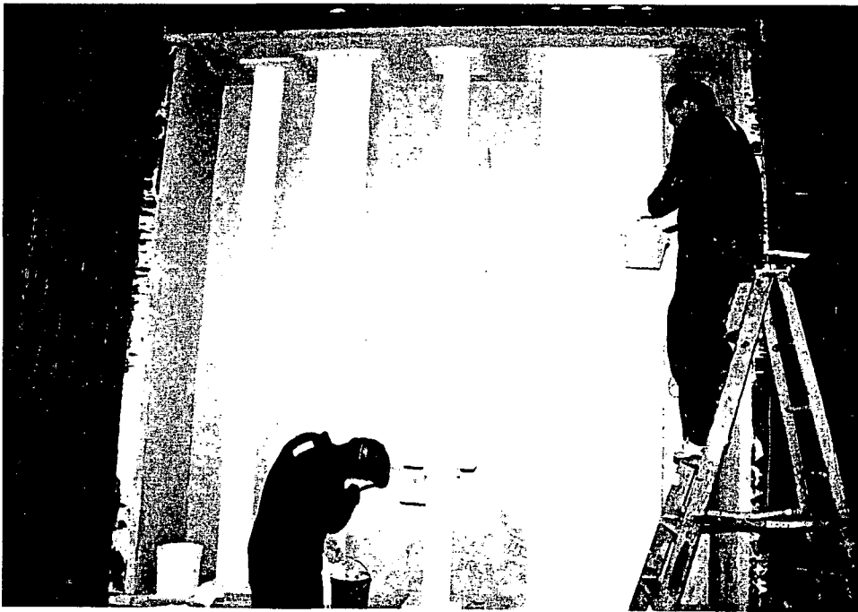
Skim coat of trowel grade material applied over all external stress skin.
