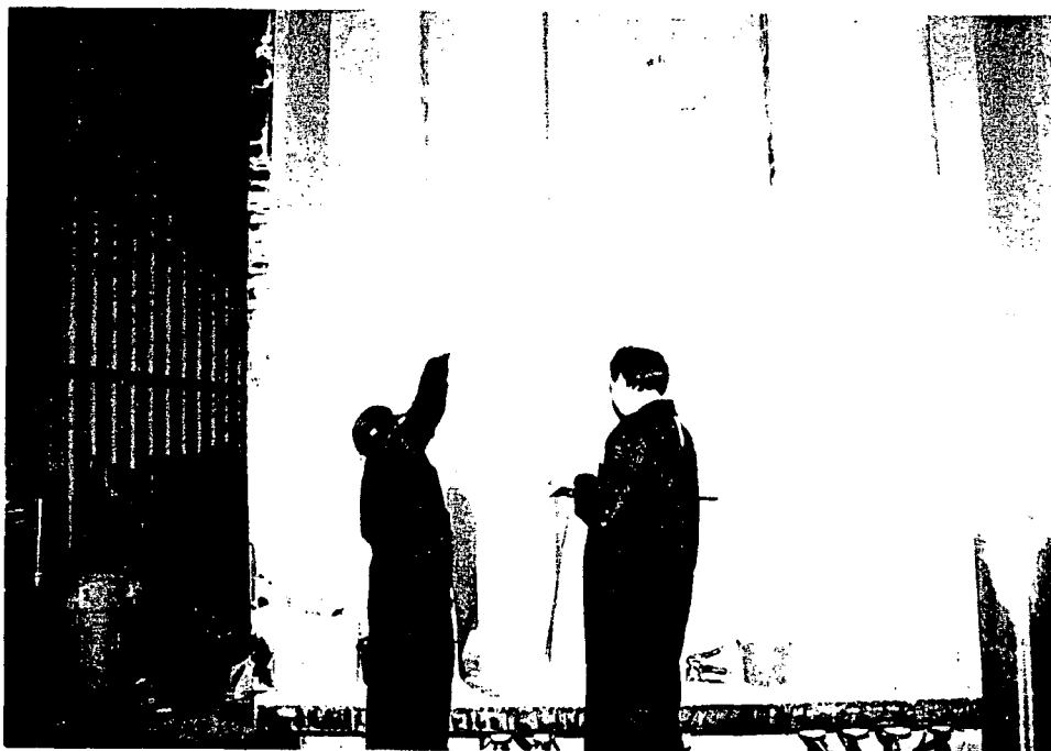
3 in. conduit enclosure wrapped with external stress skin.
