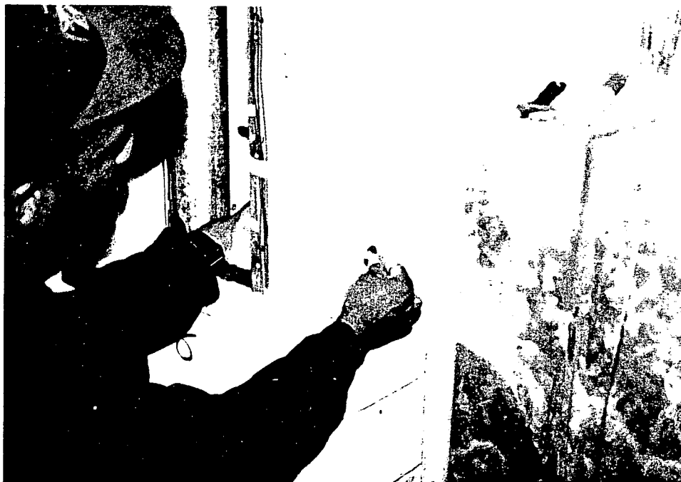
Panels secured at joint location with threaded rod, washers and nuts.
