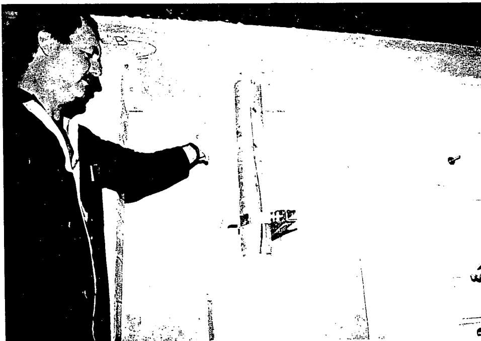
Pre-shaped conduit sections installed on conduit above junction box.
