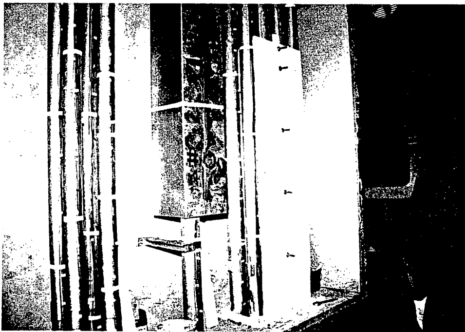
Panel secured with threaded rod, washers and nuts.
