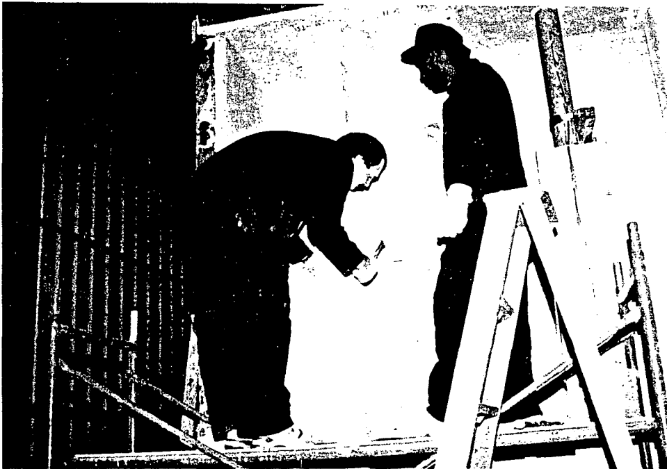
Panels secured with stainless steel tie wire.
