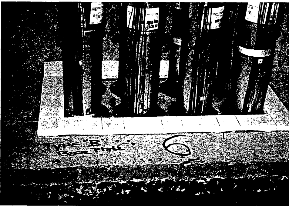
Base plate material mocked-up on bottom of set of 4 in. conduits.
