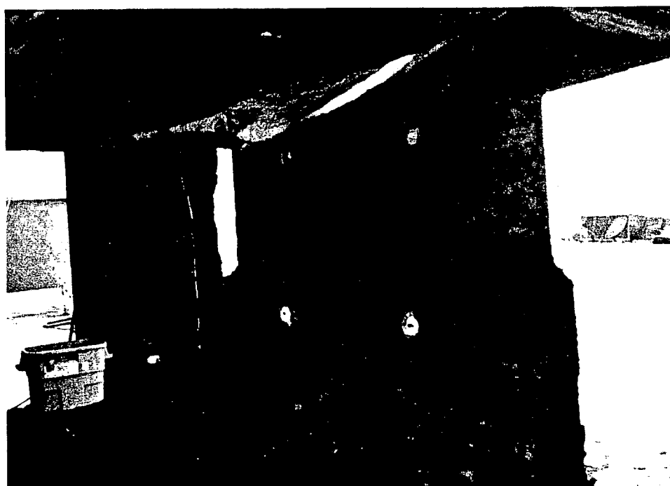
Trowel grade mounds removed from panel.
