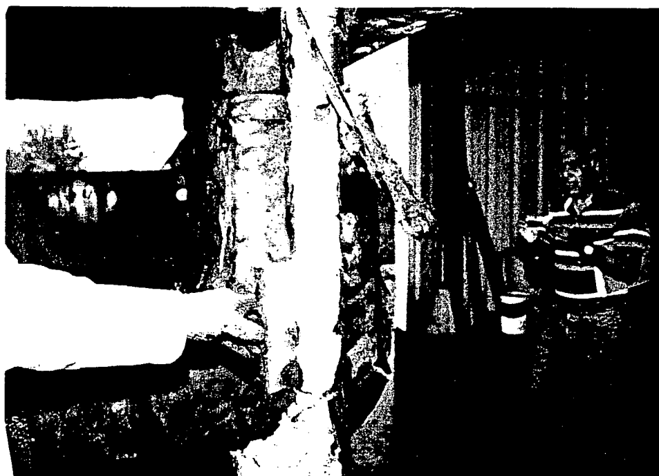
Outer layer of material removed from left 3/4 in. conduit above radial bend.
