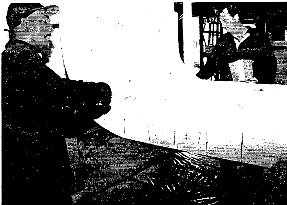
Skim coat of trowel grade material applied to enclosure.
