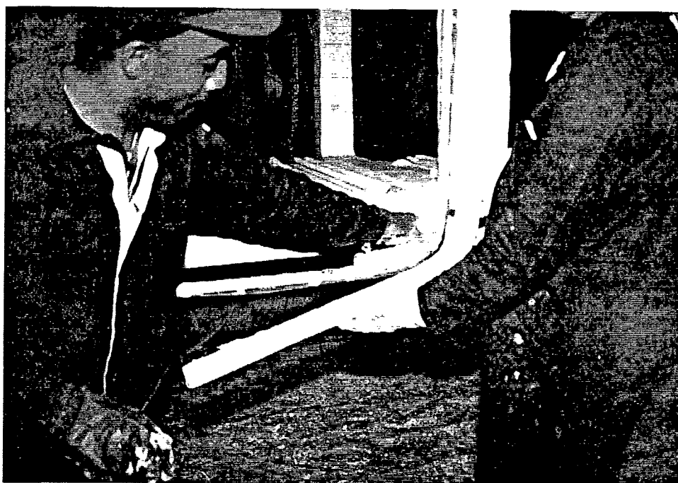
Pre-buttered pre-shaped conduit sections installed on radial bend.
