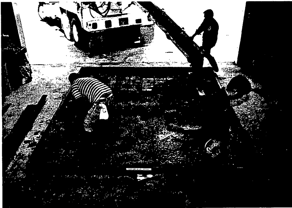
Pouring concrete into steel form for deck.
