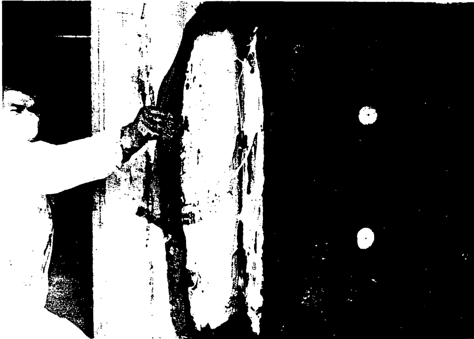
Material removed from left side of junction box.
