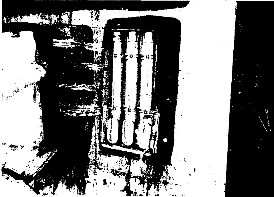
Interior of lower conduit bank enclosure.
