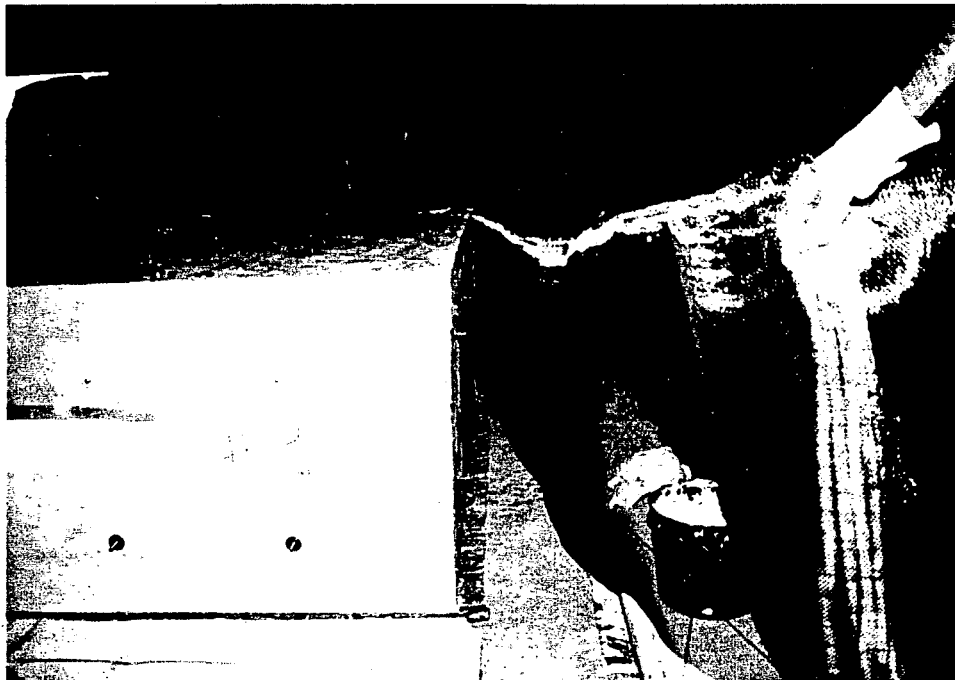
External stress skin wrapped around side of junction box enclosure.
