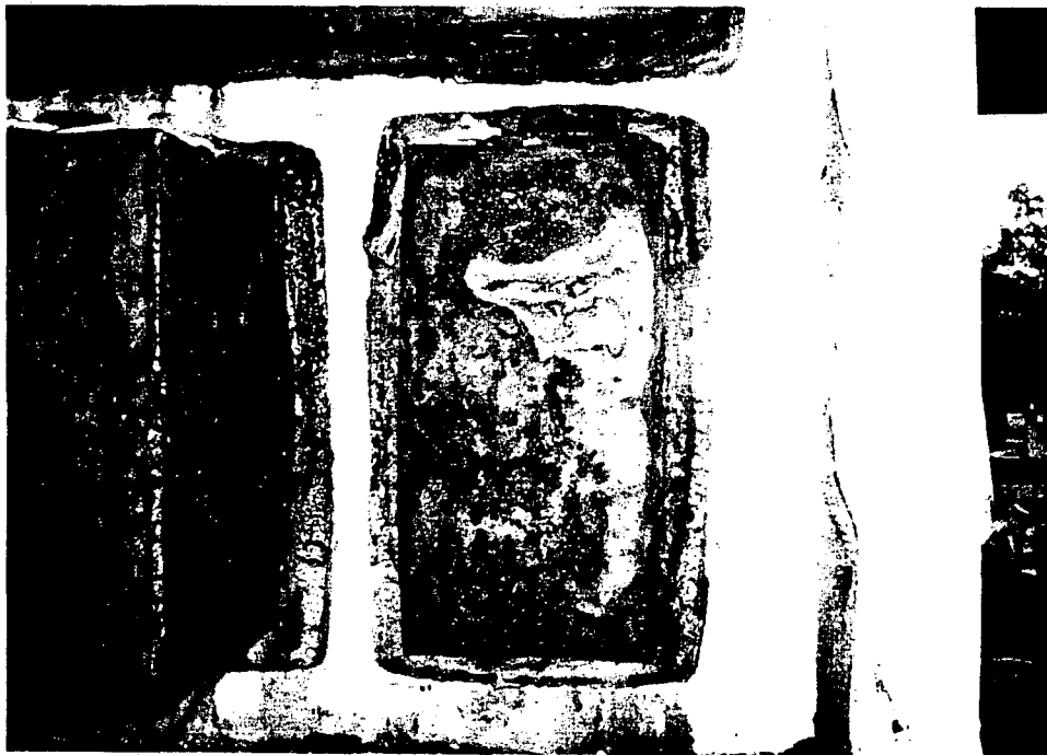
Lower conduit bank enclosure after hose stream.
