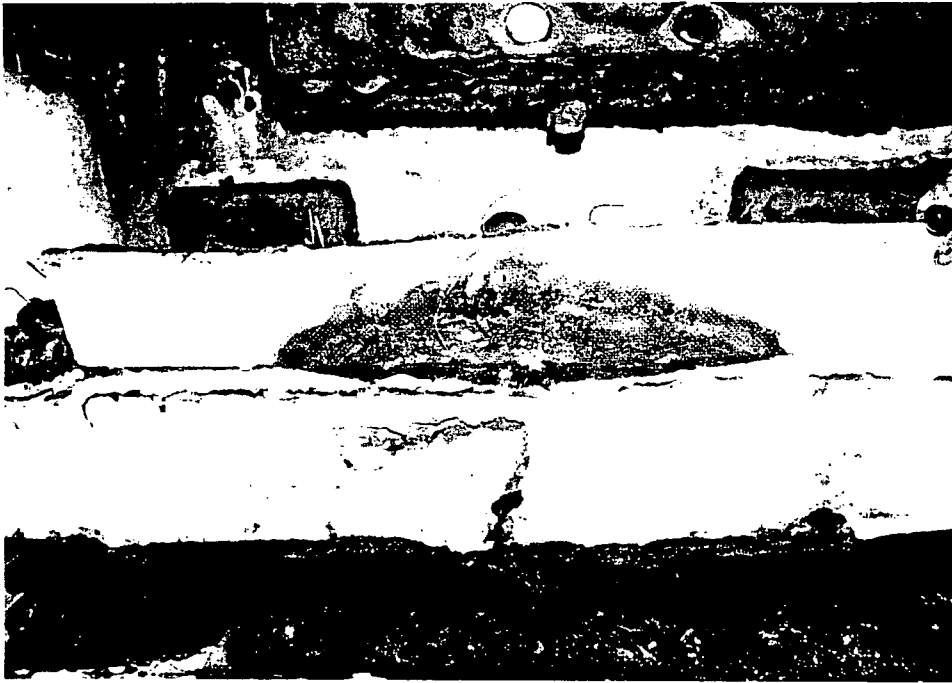
Material removed from rear of bottom bar of right support (bare tray on bar).
