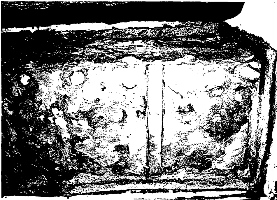
End of large enclosure after water hose stream.
