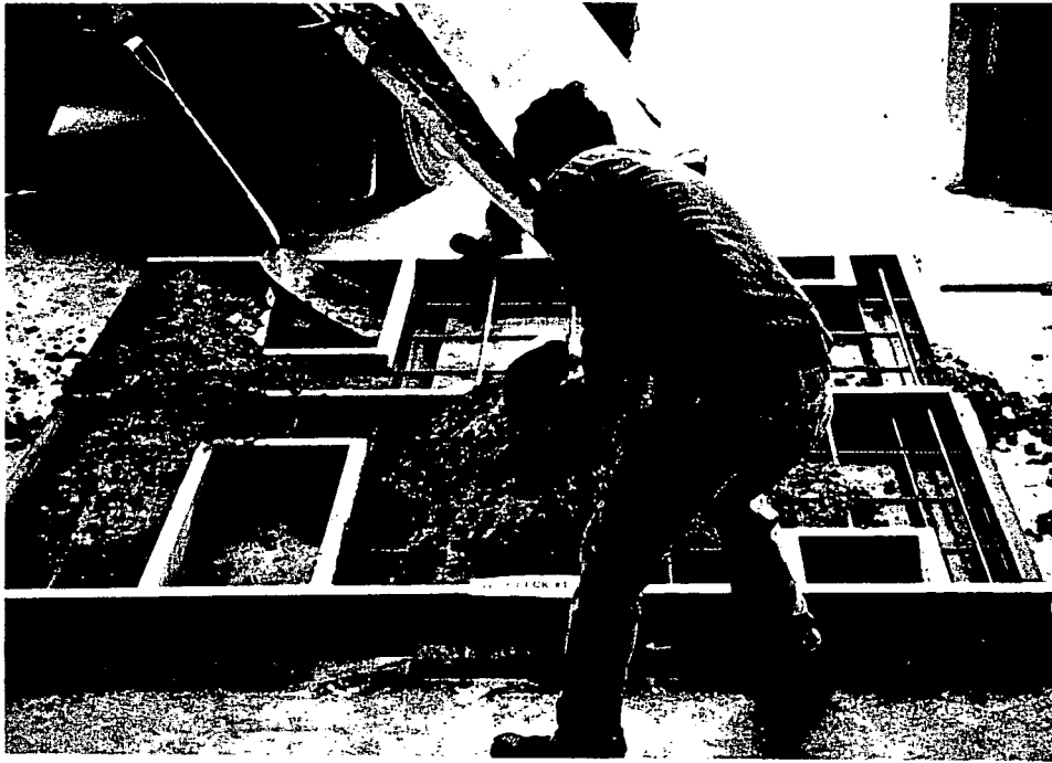
Pouring concrete into steel forms for deck end walls.
