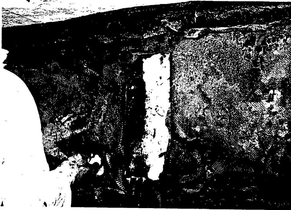
External stress skin removed from small enclosure.
