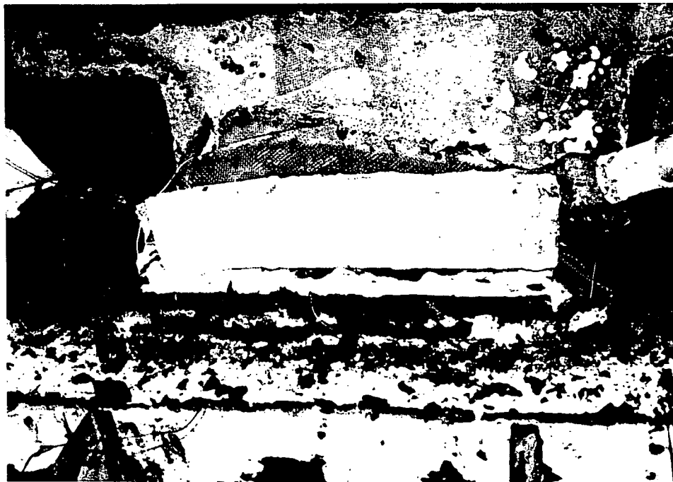
External stress skin and panel removed from rear of center, wrapped tray of right support.
