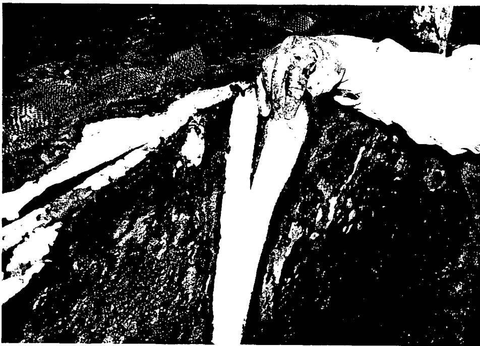
Strip removed from joint on bottom of large enclosure.
