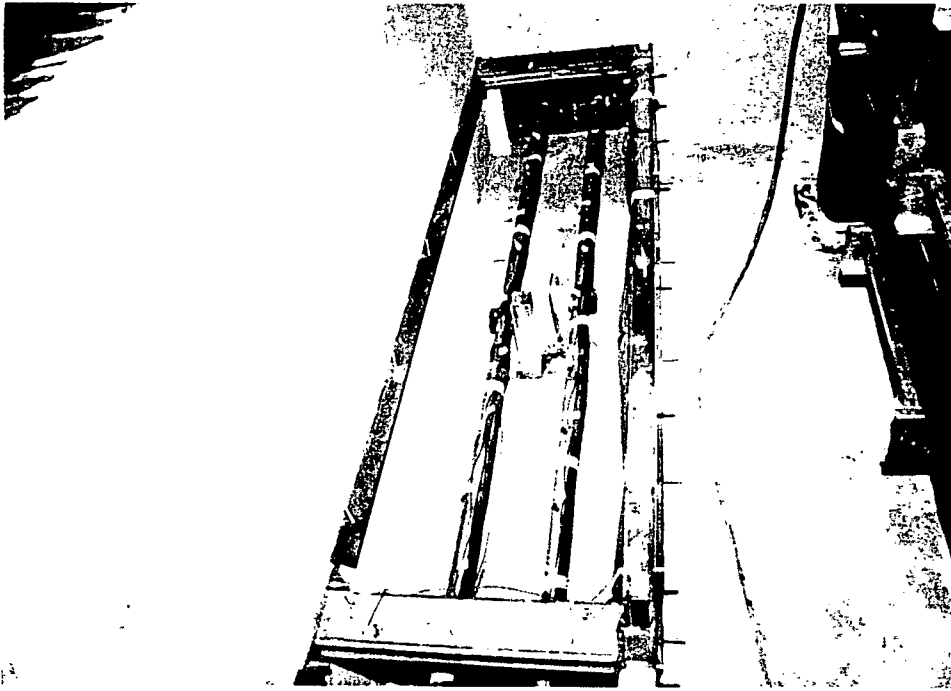
Small two-sided enclosure frame with two 1 in. steel conduits.
