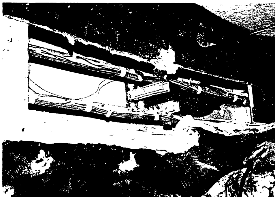
Interior of small enclosure.
