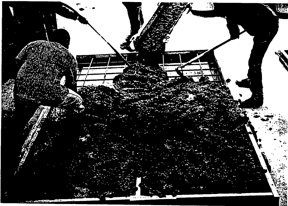
Pouring concrete into steel forms for deck side walls.
