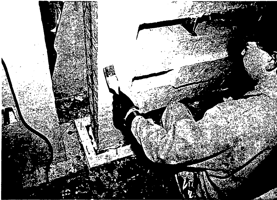
Skim coat of trowel grade material smoothed with a wet brush.
