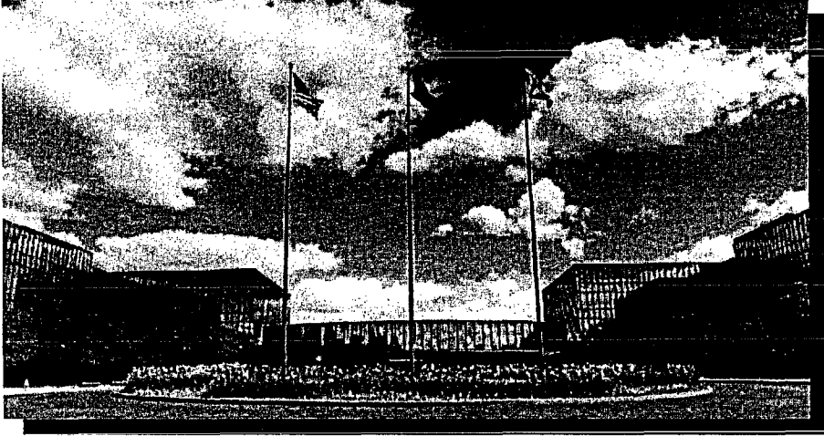
Westinghouse Electric Company Headquarters Energy Center, Monroeville, Pa, USA
