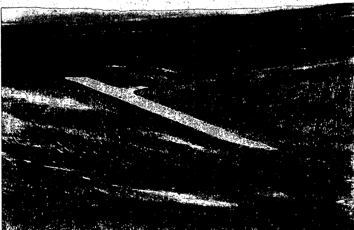
SBS 6/2007. PL-7. Riprap-armored drainage feature on the south flank of Pit 4.
