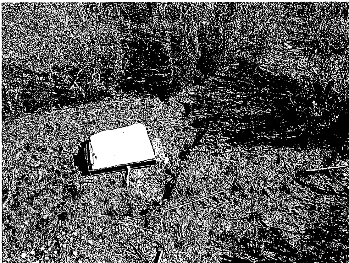
BAR 8/2007. PL-5. Cracks in the tailings impoundment cover soil near erosion monitoring point C2.
