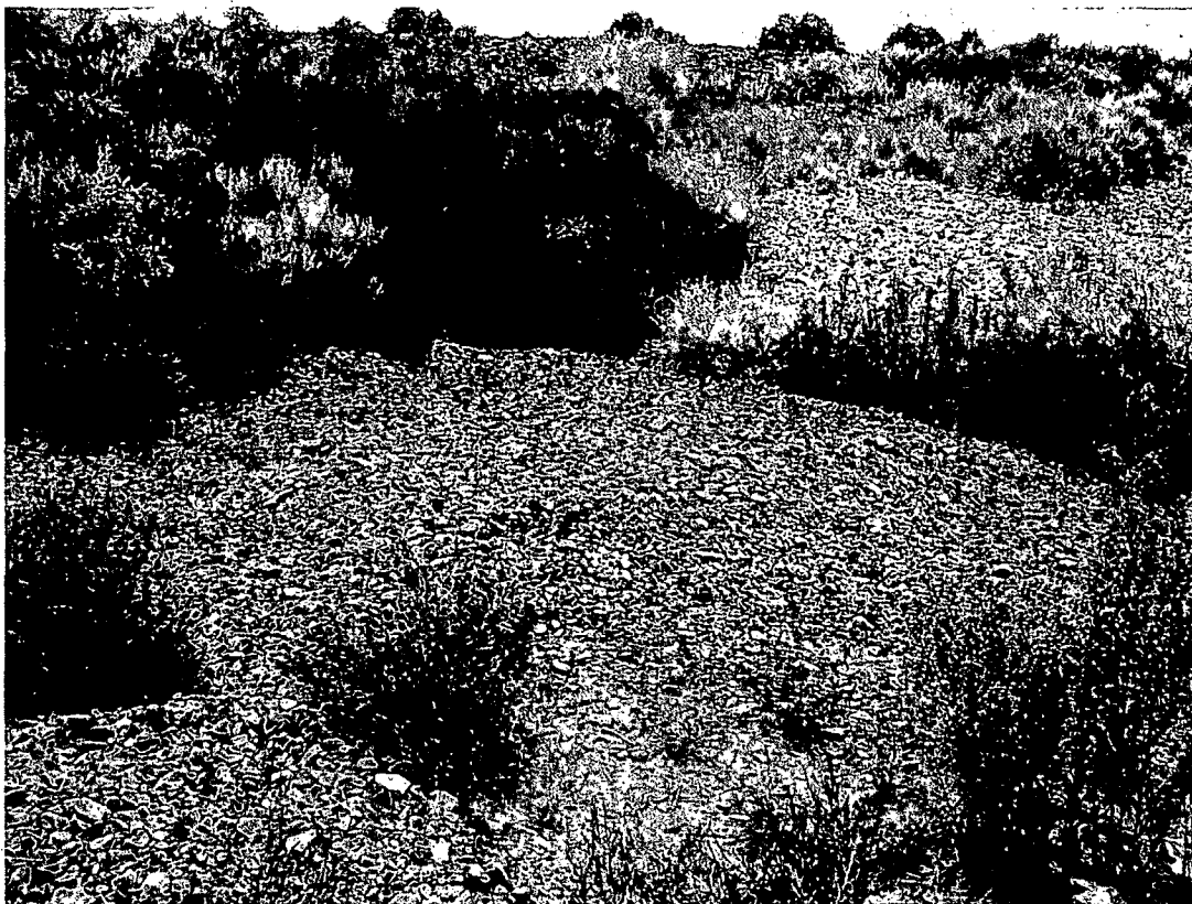
BLU 8/2007. PL-7. Repaired depression in the asbestos disposal cell cover.
