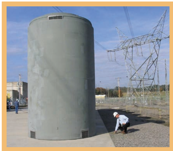
Scott Atwater, Region IV DNMS inspector, checking dry fuel storage casks at Arkansas Nuclear One in Russellville, AR
