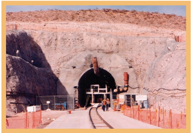
Yucca Mountain Tunnel Entrance, Eureka County, NV
