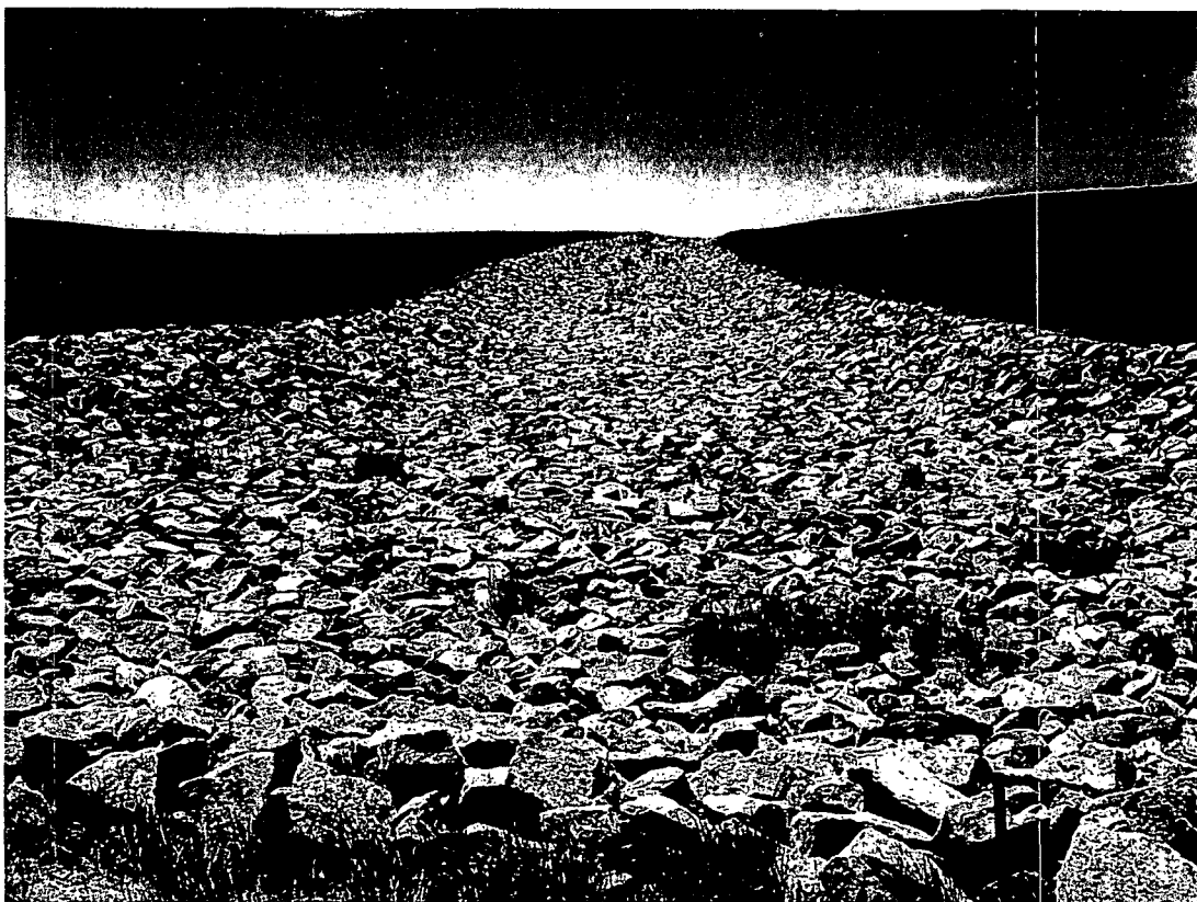
SBS 6/2007. PL-6. Rock-armored erosion control structure west of the disposal cell.
