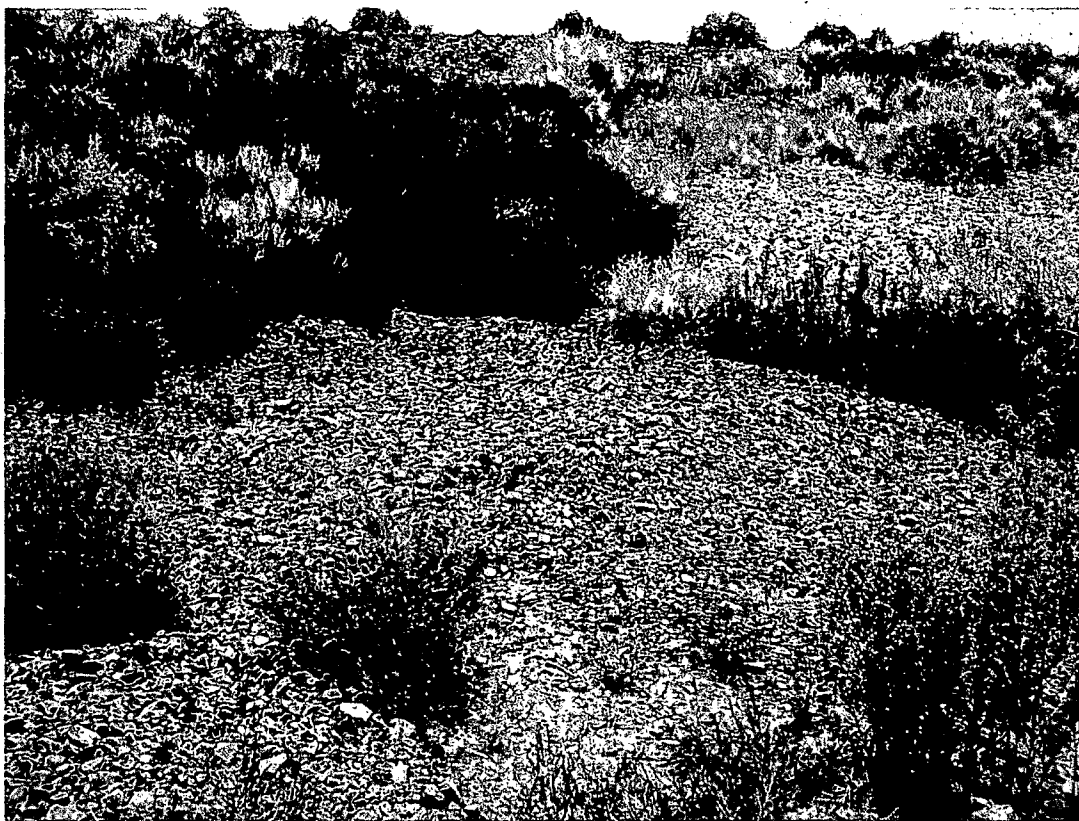
BLU 8/2007. PL-7. Repaired depression in the asbestos disposal cell cover.
