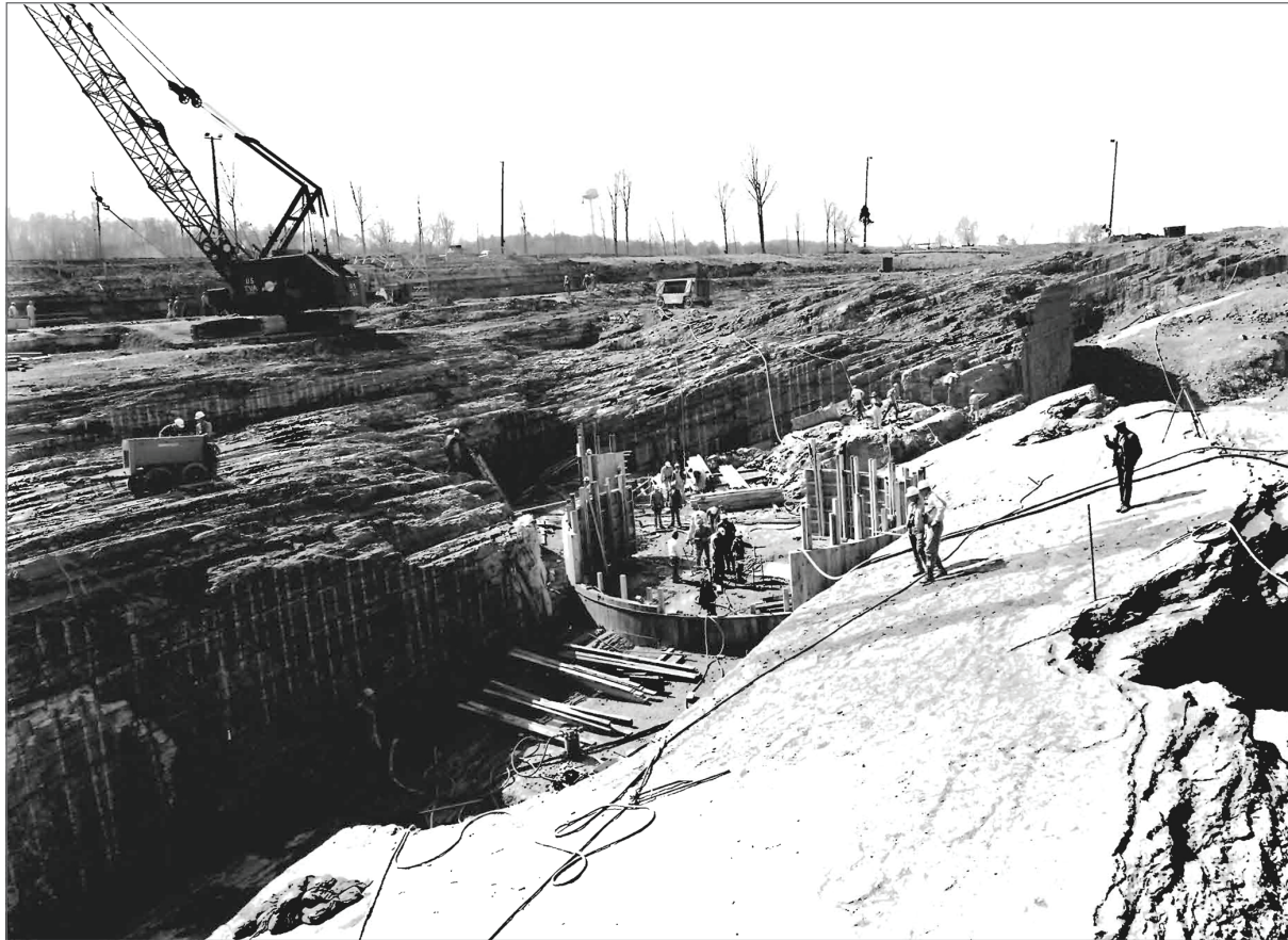
1975 Excavation for Unit 1 reactor, showing dipping beds of hard, fresh limestone
