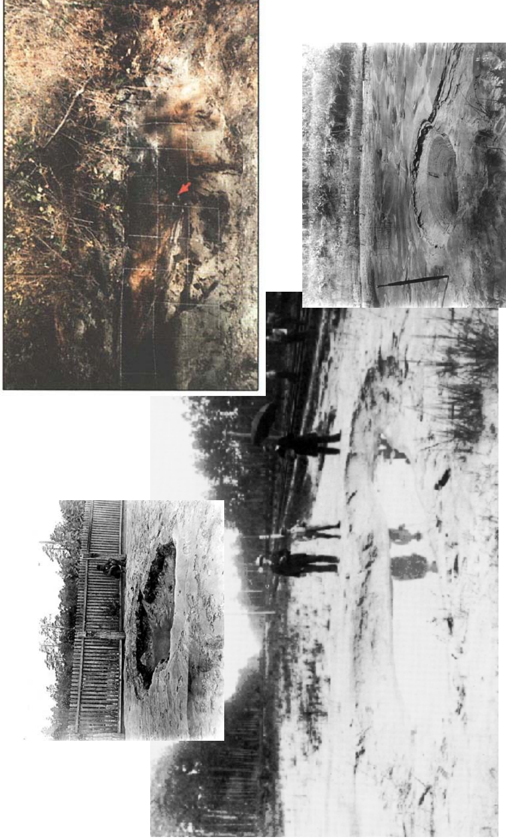
Illustrations of historic 1886 liquefaction features from the Charleston Area
