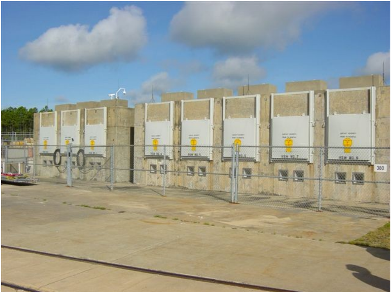
H. B. ROBINSON STEAM ELECTRIC PLANT, UNIT NO. 2, INDEPENDENT SPENT FUEL STORAGE INSTALLATION
