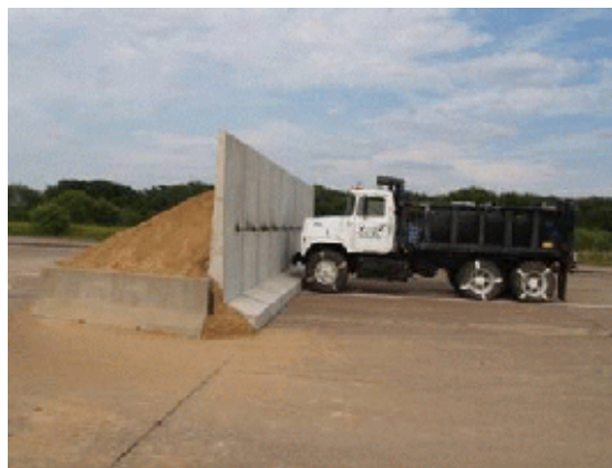
Figure 5-6. Concrete and sand vehicle barrier
