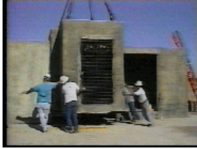
Figure 5-55. Silent Defender® module delivered to site.
