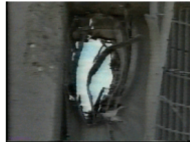
Figure 5-59. Hole resulting from use of explosives on Silent Defender®.
