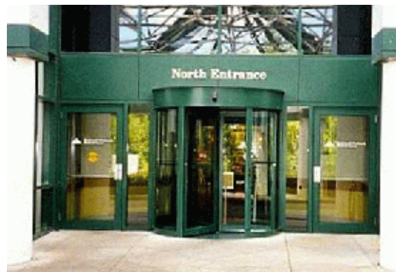
Figure 5-37. Commercially available access control revolving door system.
