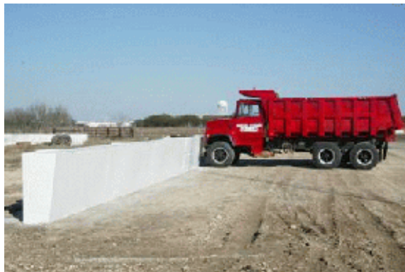
Figure 5-8. RSA vehicle barrier.
