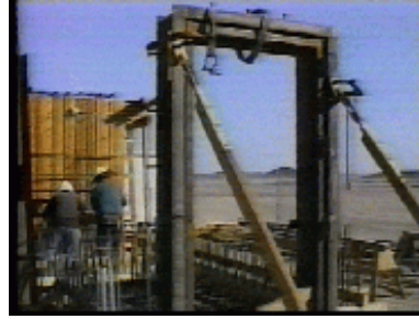
Figure 5-56. Silent Defender® module being constructed on site: door frame placement.
