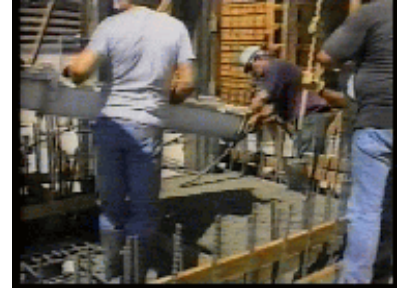
Figure 5-57. Silent Defender® module being constructed on site: concrete pour.
