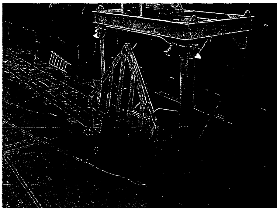
Figure 4-8 Trash rake and trash cart apparatus at the Dilution Water System (top) and the Circulating Water System (bottom) intakes. Note floodlights attached to trash carts.
